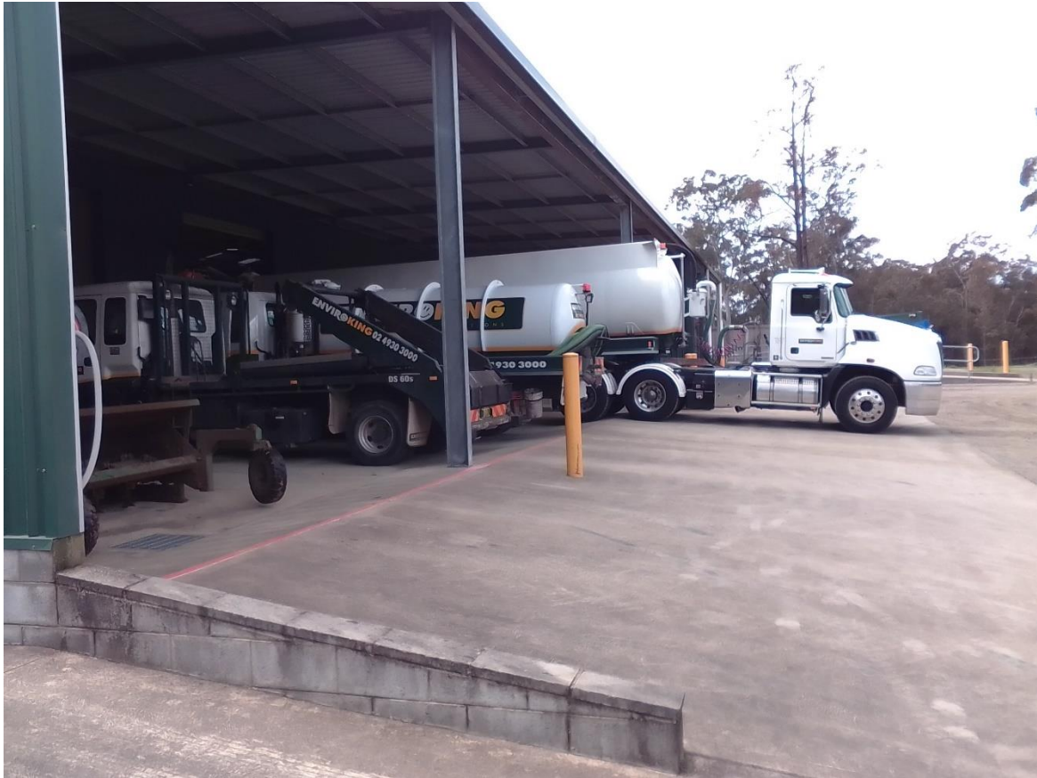
Plate 11 Bunded vehicle parking location
