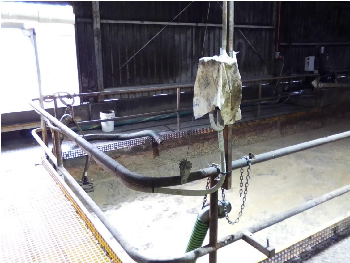
Plate 9 Internal Grease Trap Sludge Pit
