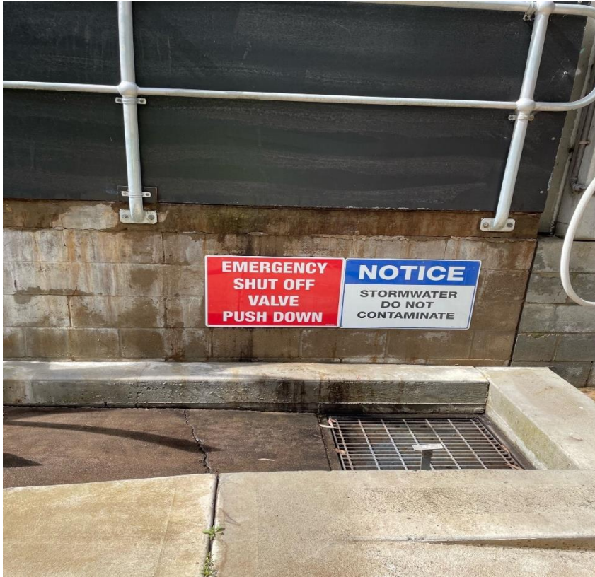
Plate 7 Storm Water Drain and Emergency Shut Off Valve
