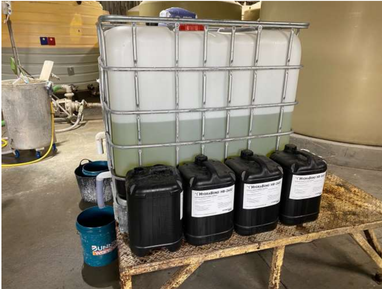
Plate 2: Chemical Storage (Alternate Angle)
