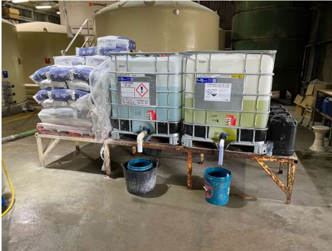
Plate 1: Chemical Storage Area
