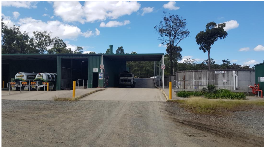
Figure 4 Receiving driveway where vehicles park under the awning on the eastern (right-hand) side of the building and pump out the collected wastes into the receiving pit.
