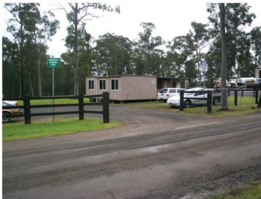
Photo 3 - Office building and employee car park.
