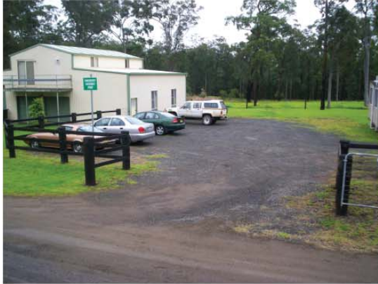
Photo 1 - Site shed and employee carpark.
