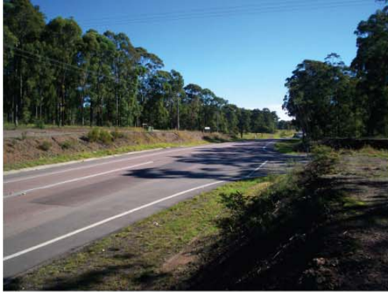
Photo 1 - View west across driveway entrance.
