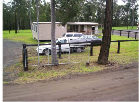
Photo 2 - Office building and employee car park.
