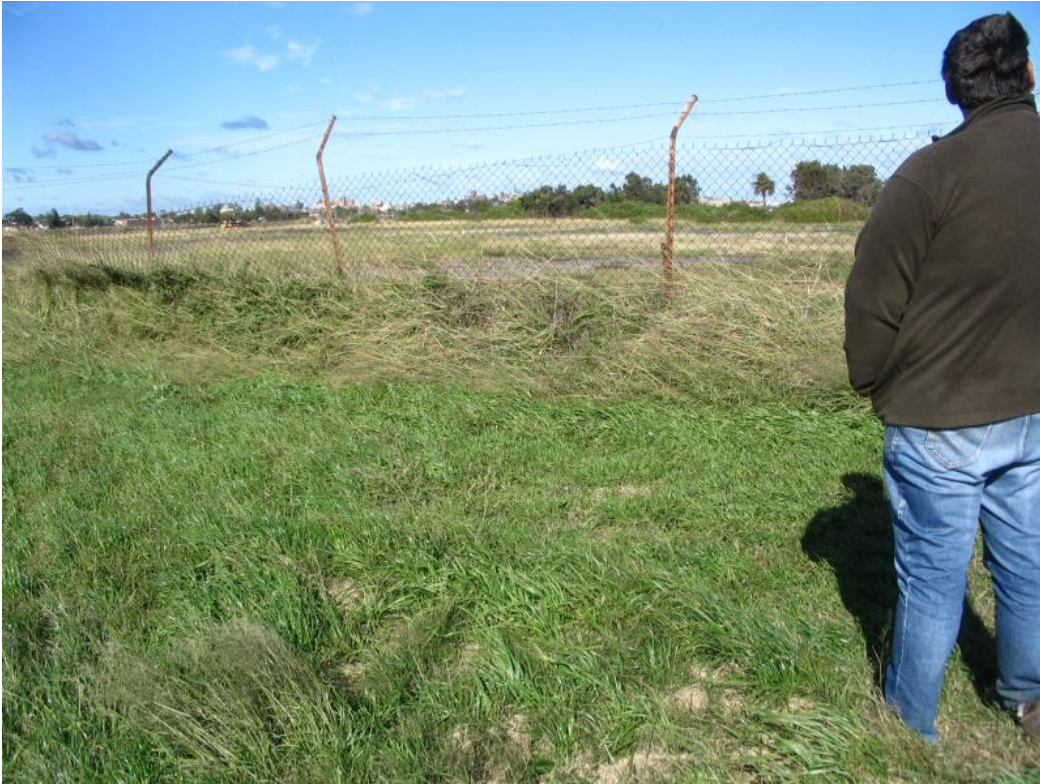
Plate 11: Dilapidating Cyclone Fence surrounding DP1 and DP2
