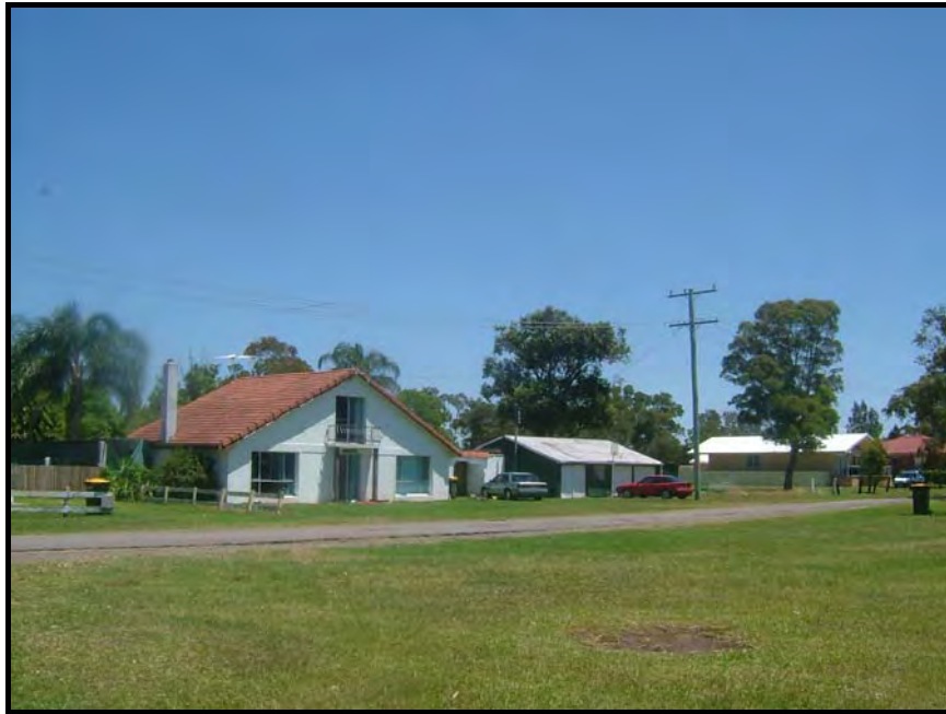
Photograph 1: View of the existing residence looking from the reserve on the eastern side of Waterfront Road.
