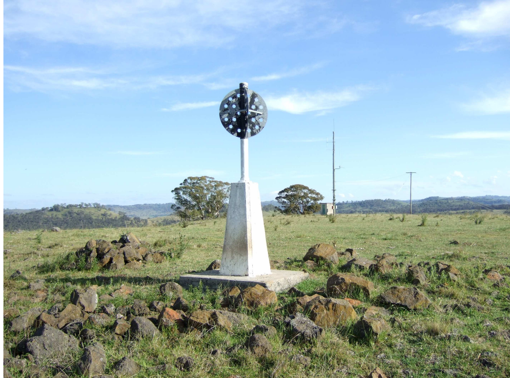
Plate 12 - Turbine Site T7 between Trig Station and NPWS radio mast in the distance On T7, native Spear-grasses Austrostipa spp. and Saffron Thistle Carthamus lanatus are also common. There are two Ribbon Gum Eucalyptus viminalis trees near T7 but on a slope that will not be disturbed.
