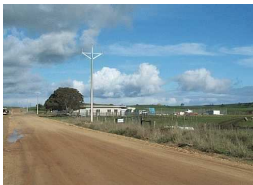
Plate 3.3 Typical Site Office and Storage Area
