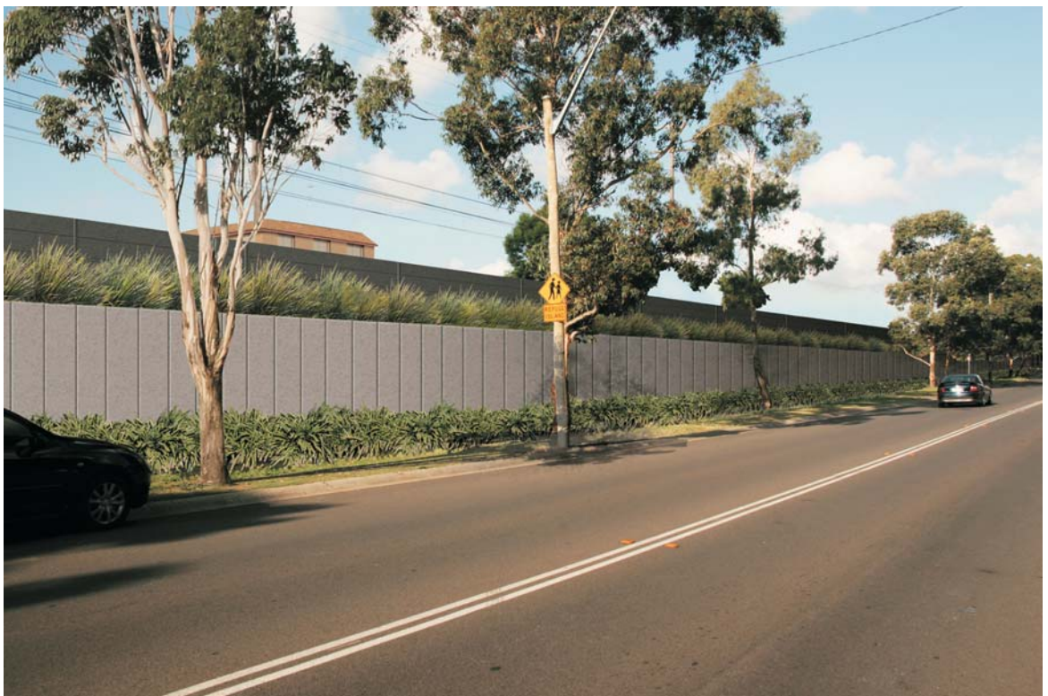
Figure 15.2 Artists impression of retaining wall along Bryant Street (noise barrier above)
