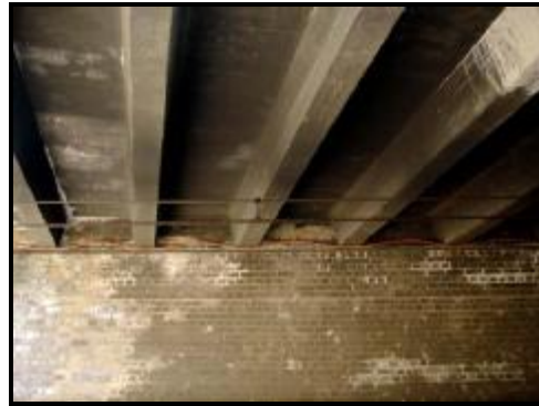
Figure 4 The original jack arch construction at Beverley Hills station has been concealed by concrete protection.
