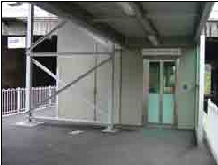
Photograph 13: Lift on platform to the north-east of King Georges Road overbridge
