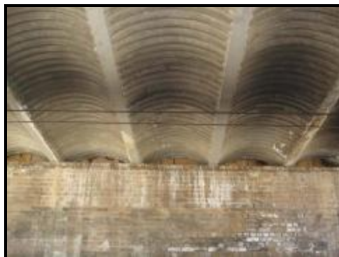
Figure 1: Jack arch construction, parallel steel beams with mini arches, usually brick, that form a working platform and support the road-fill material Figure 2: Two-span overbridge at Padstow.
