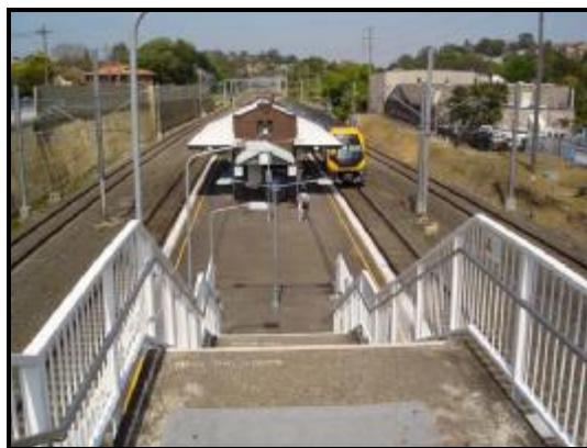
Figure 7 A symmetrical platform at Turrella station.
