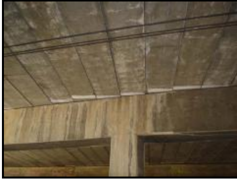
Figure 5 Concrete construction for the Northbound carriageway at Beverly Hills.
