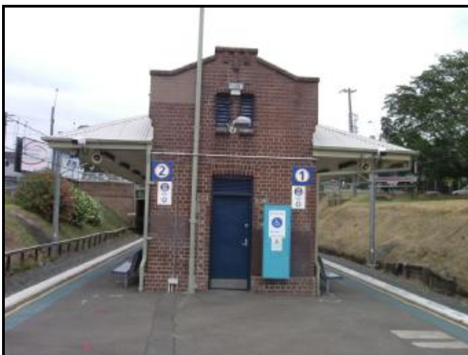
Photograph 9: View of the eastern elevation of Beverly Hills Railway Station building.
