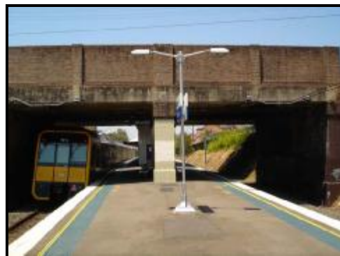
Figure 1: Jack arch construction, parallel steel beams with mini arches, usually brick, that form a working platform and support the road-fill material Figure 2: Two-span overbridge at Padstow.
