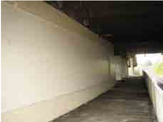
of King Georges Road overbridge to be demolished
