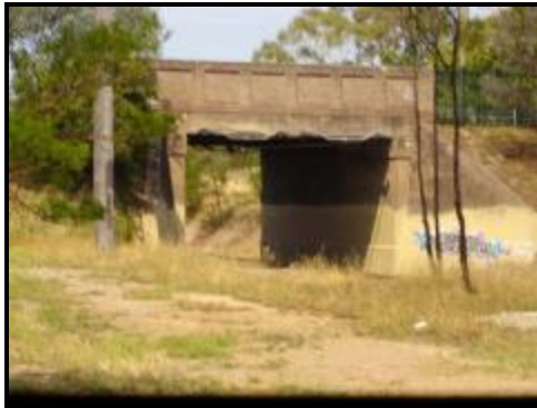
Figure 3 Single span jack arch overbridge for Park Rd, Panania.
