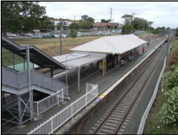
Photograph 5: Beverly Hills Railway Station from the overpass.
