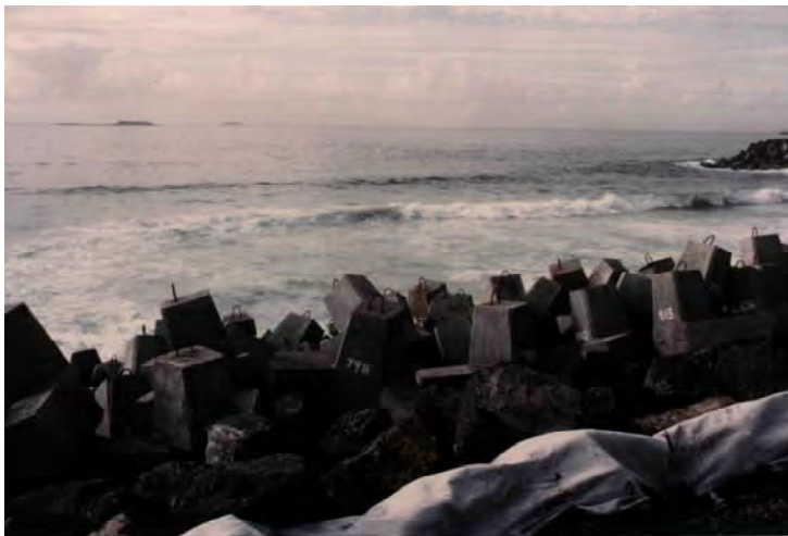
Hanbars & Rock placed directly on ELCOMAX® geotextile
