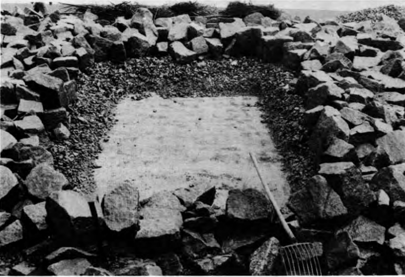
Fig. 6. Needle-punched nonwoven fabric after removing the revetment cover layers.
