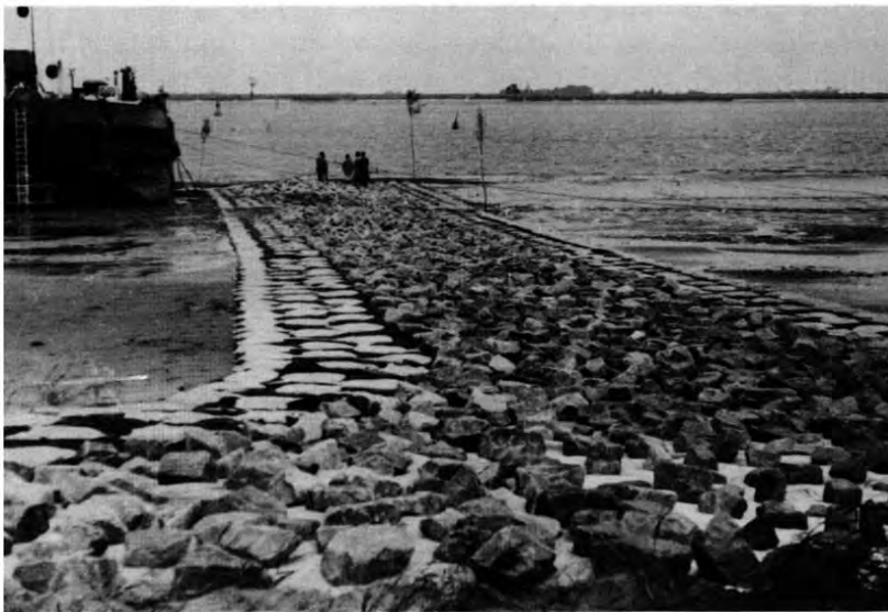
Fig. 16. Groin at the River Weser: under construction at tidal low water.
