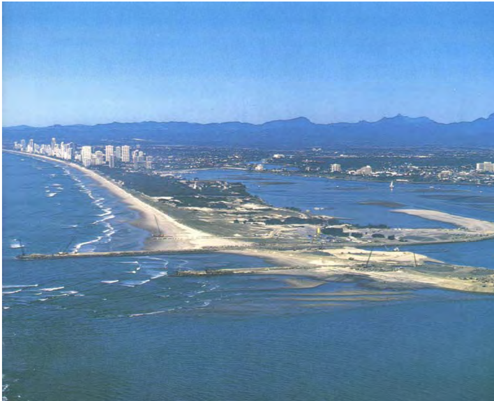
Training walls under construction 1985
