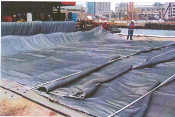
Rebar and prep/staging | The rebar was attached approximately every 10 yards along the length of the fabric to help in deploying fabric into the water and to aid in positioning the fabric on the seafloor. Photo courtesy of Triumph Geo-Synthetics.
