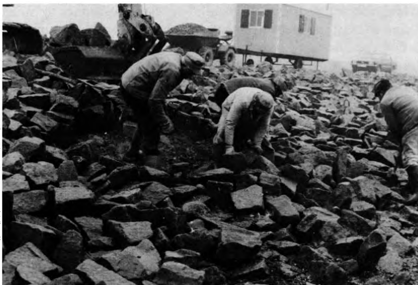
Fig. 5. Sampling operations at the seadike revetment.
