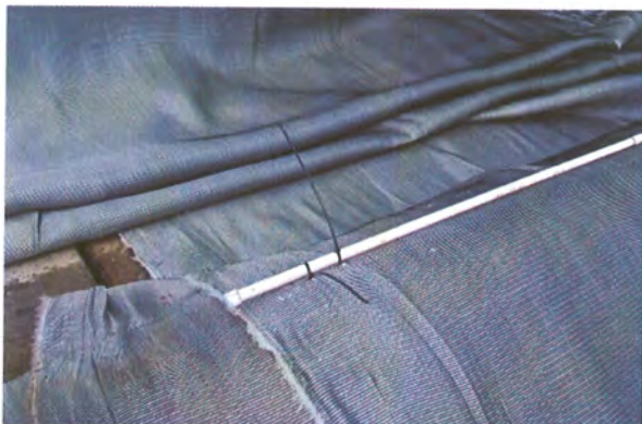
Rebar and prep/staging | The rebar was attached approximately every 10 yards along the length of the fabric to help in deploying fabric into the water and to aid in positioning the fabric on the seafloor. Photo courtesy of Triumph Geo-Synthetics.
