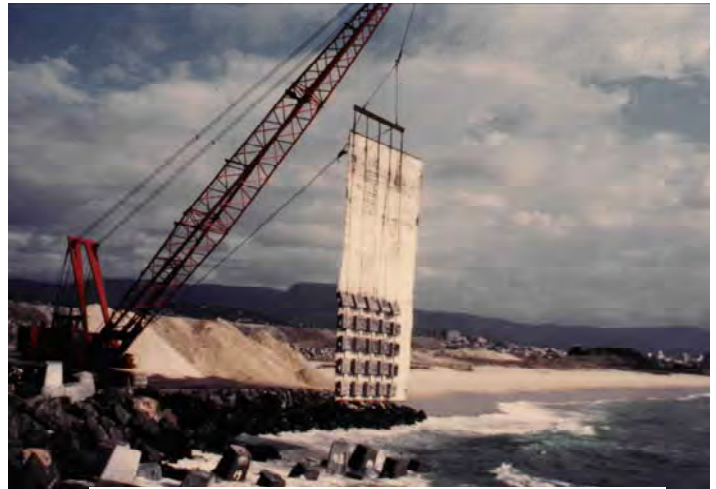
Installation of ELCOMAX® 1200R
