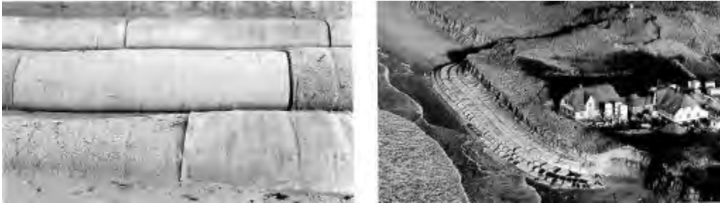
Figure 3: Protection of an artificial dune near Kampen (Island of Sylt, Germany) by a light geotextile revetment
