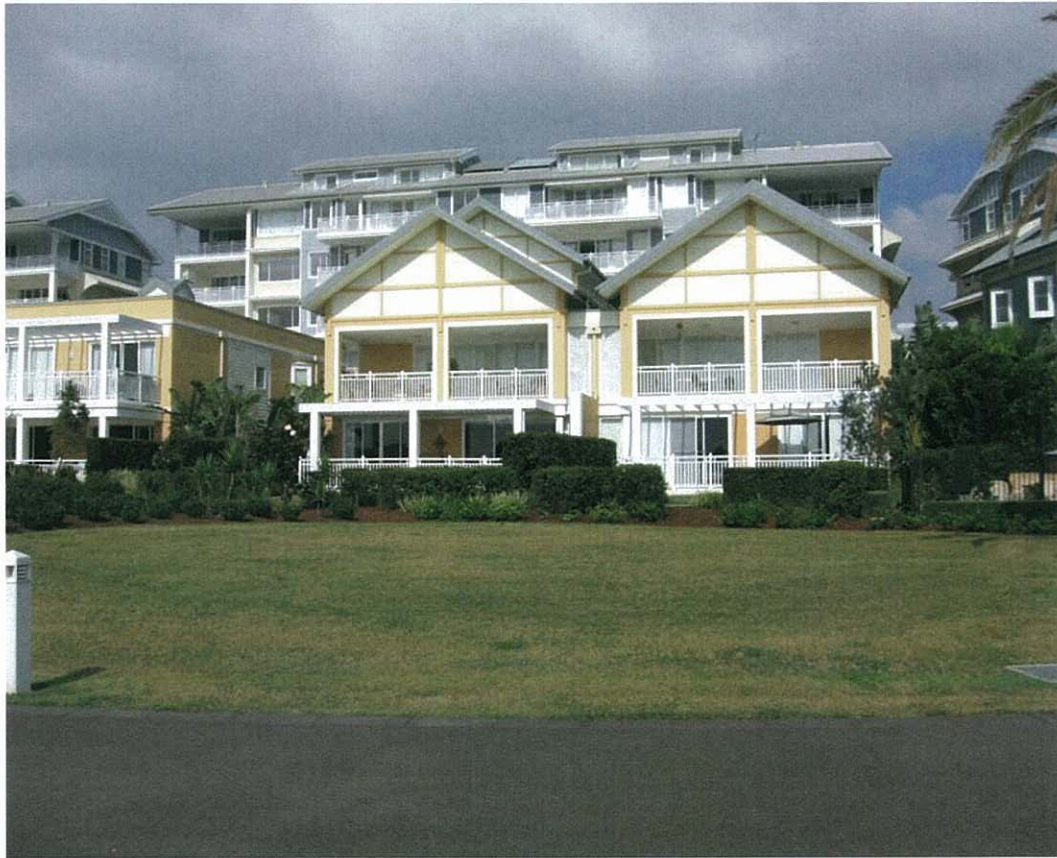
From seawall. Hunters Wharf with walkway in foreground. Note extensive use of glass and the proximity of the walkway. See comment under Attachment 26.
