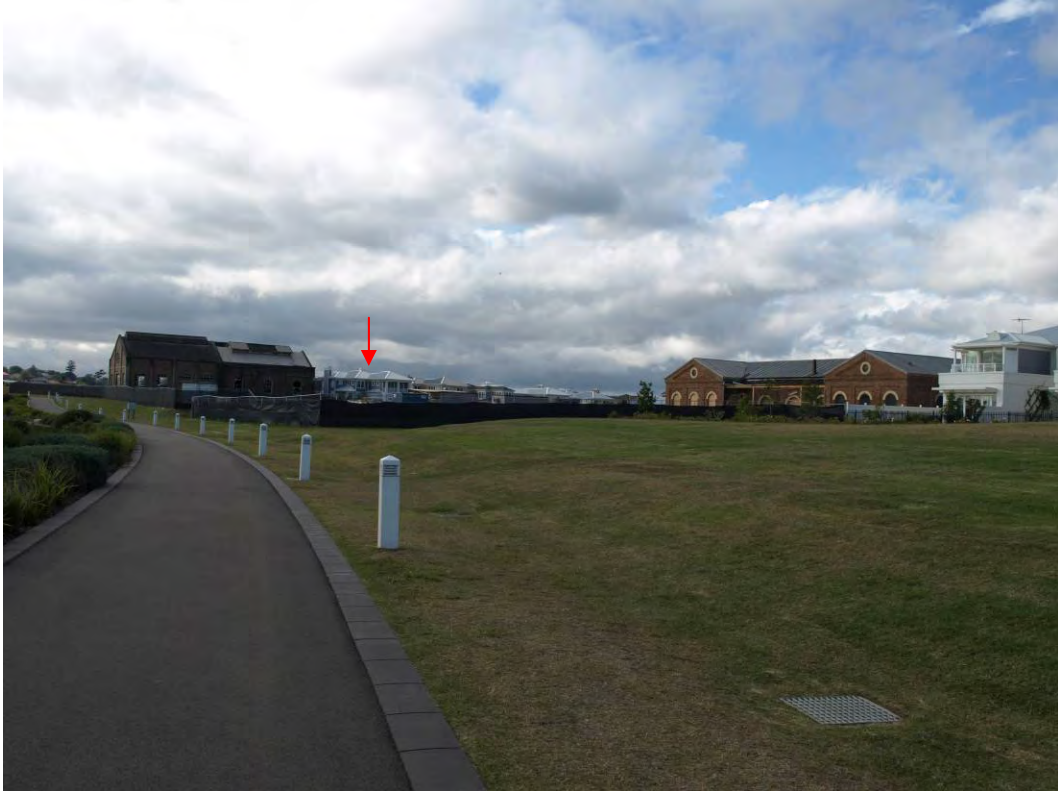
Plate P7: View of the Former AGL Blacksmiths' Workshop (right of image) towards site of proposed Marina (approximate location marked with arrow).
