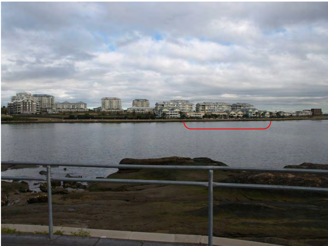
Plate P8: View from Cabarita Point towards the Former AGL Powerhouse with the site of the proposed Marina to the left of image (approximate location in bracket).
