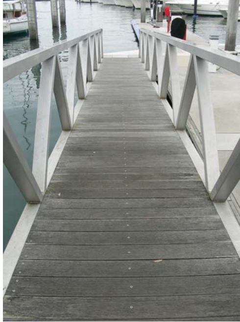
Photograph 13: Ramps – View along Aluminium Access Ramp with Timber Deck.
