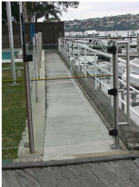
Photograph 12: Gates – View of Glass Security Gate.
