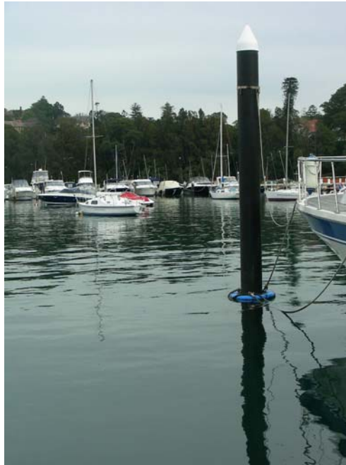
Photograph 9: Piles – View of Mooring Pile with HDPE Sleeve. Photograph taken at low tide.
