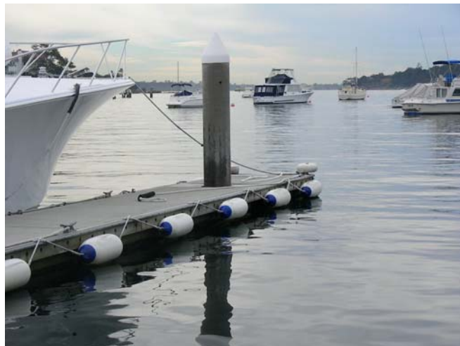
Photograph 4: Floating Structure – View of Seaward End of Concrete Type Finger with Concrete Pile and Pneumatic Fenders.
