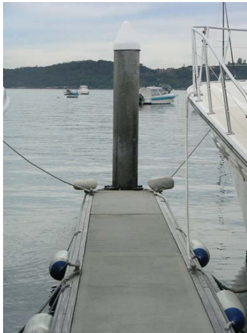
Photograph 8: Piles – View of Concrete Pile.
