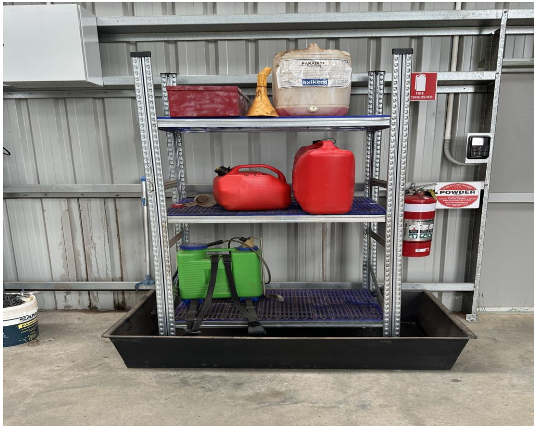
Stored chemicals with bunding
