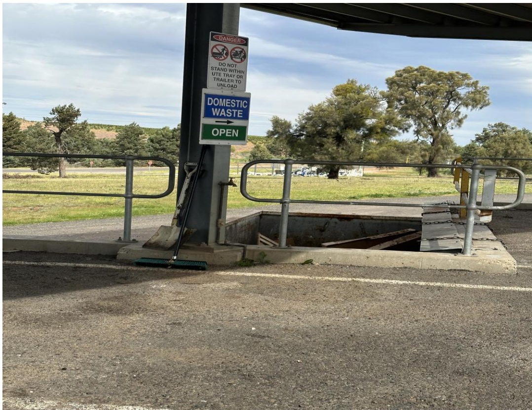
Waste transfer station domestic waste segregation area
