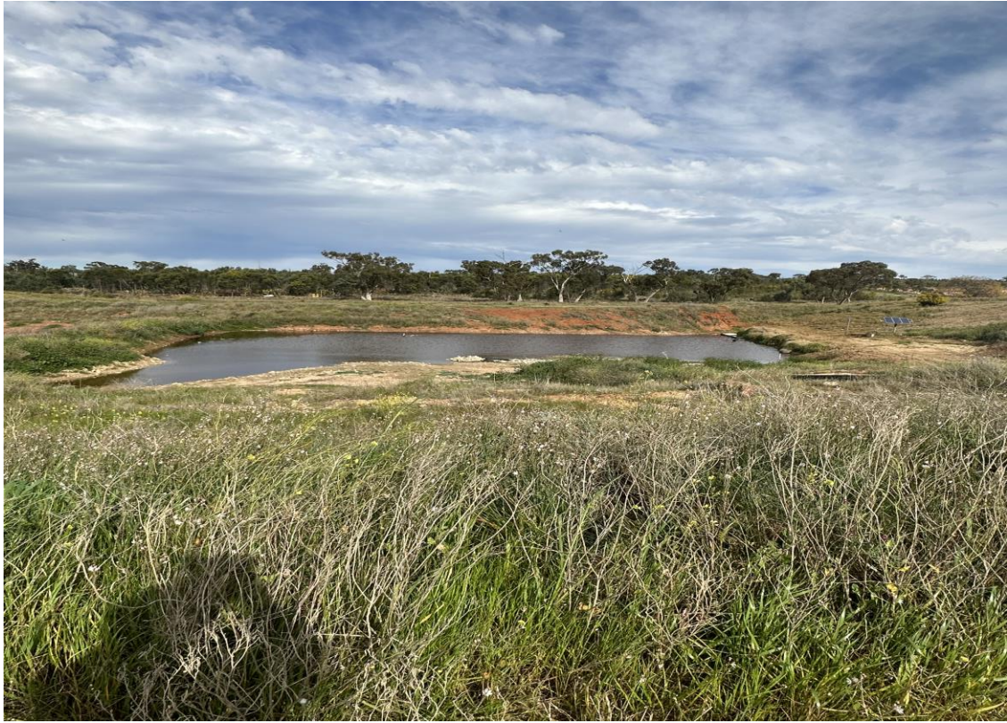
The existing leachate pond
