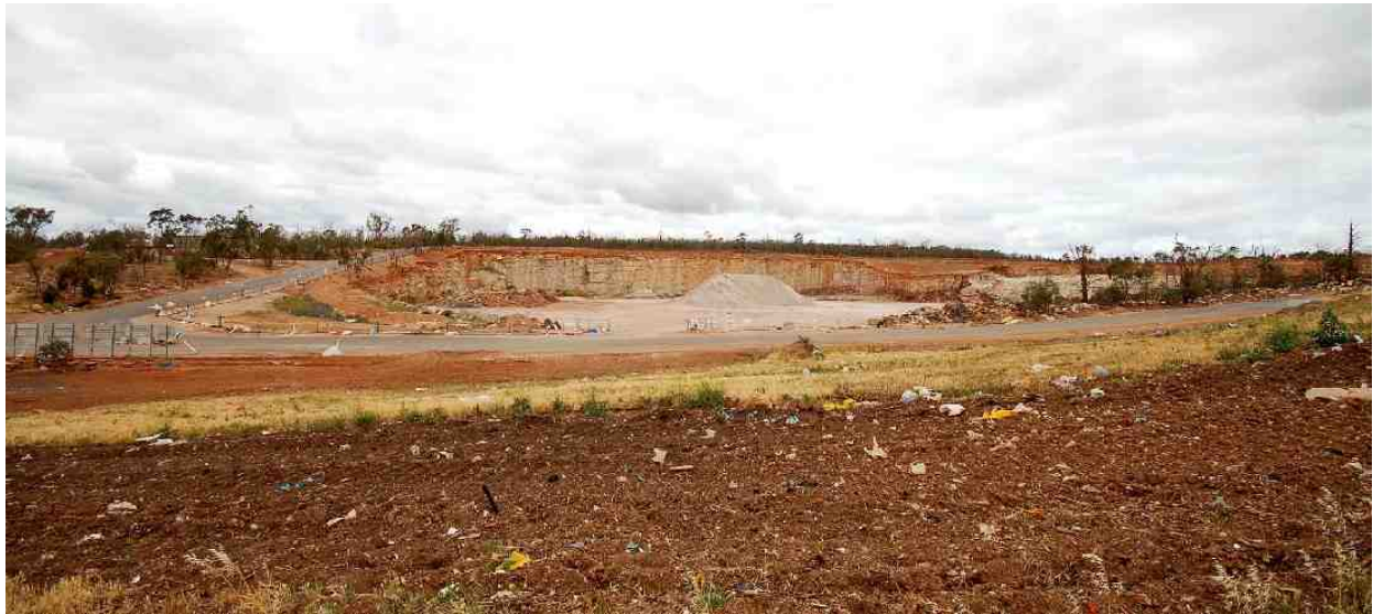
7 New soil cap over landfill (in foreground), quarry for extension of landfill in background.
