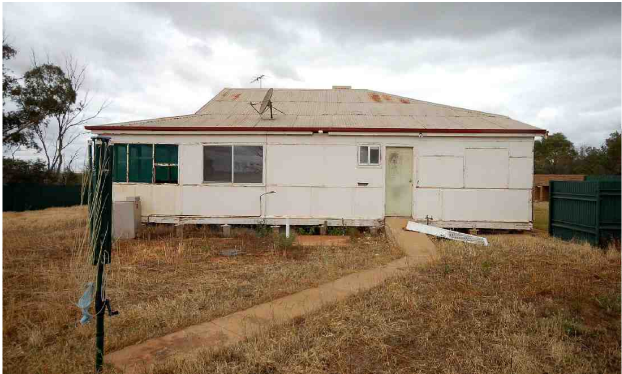
17 Caretaker's cottage, south elevation
