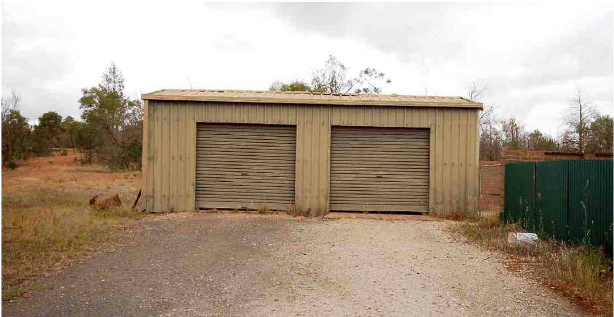
22 Caretaker's cottage, garage north elevation
