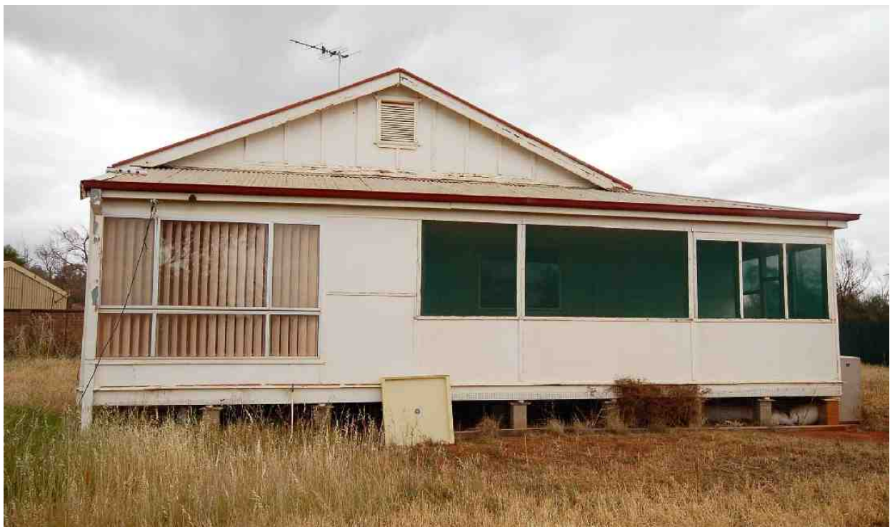
16 Caretaker's cottage, north elevation
