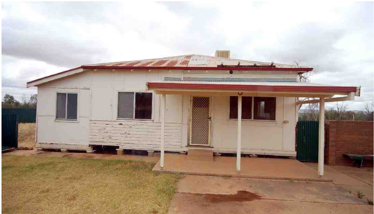
19 Caretaker's cottage, south elevation
