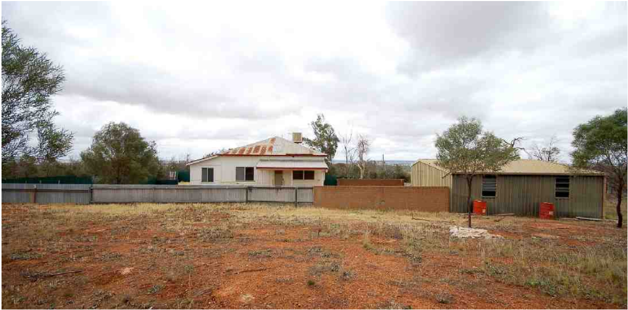
21 Caretaker's cottage, south elevation
