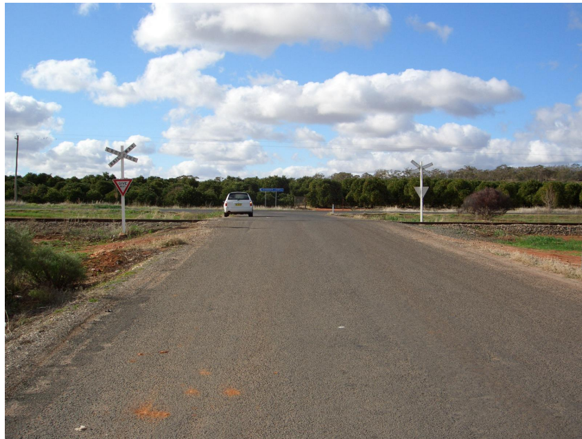
Photo 4 –Road connecting Slopes Road to Kidman Way
