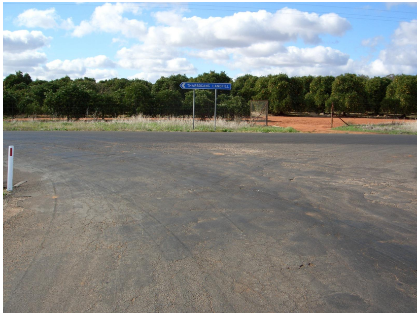
Photo 3 –Slopes Road / Access Road Intersection
