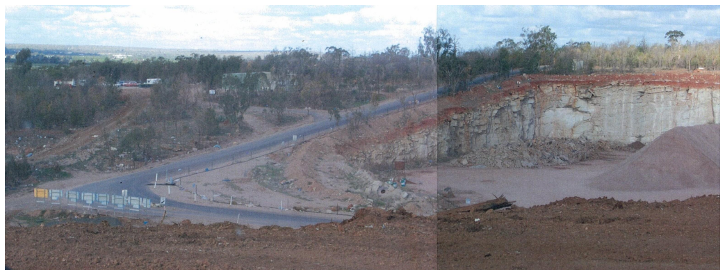
Photo 7 –Existing Site – Internal Operation
