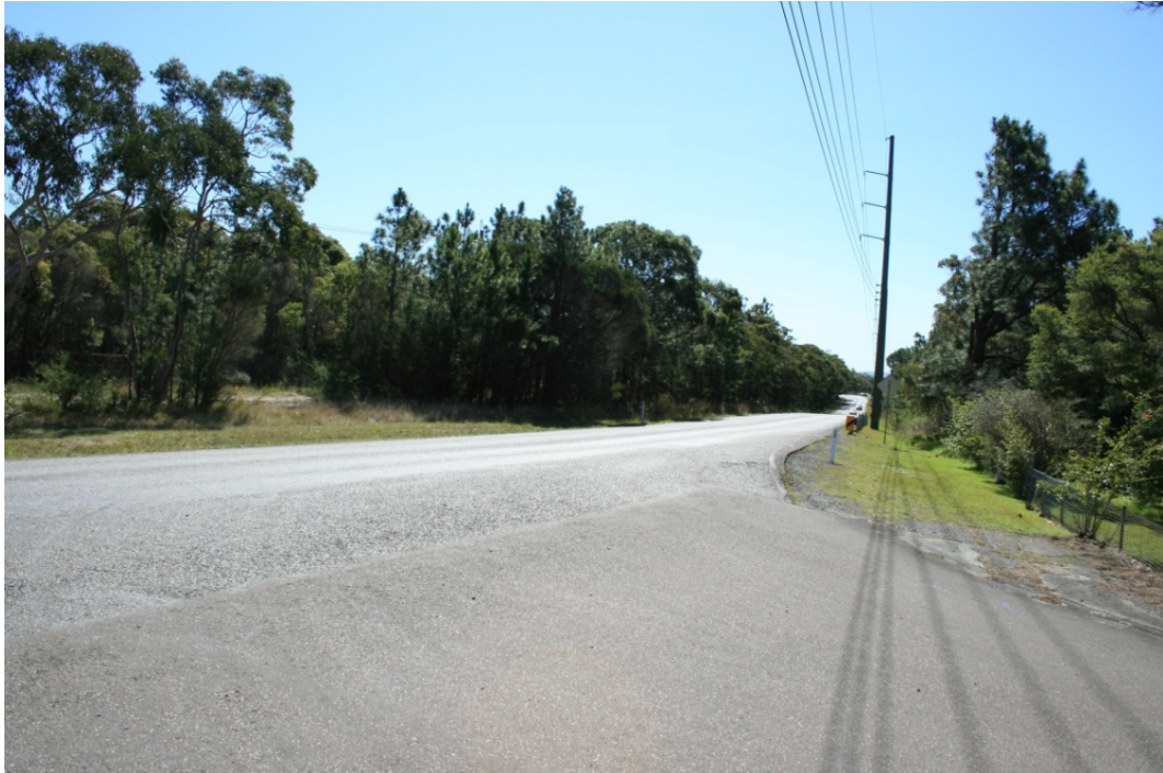
Figure 1.4 Rutleys Road, looking northbound from the intersection with Mannering Colliery Access Road
