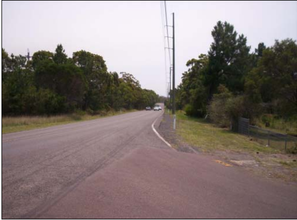
Photo 3: Rutleys Road Northbound
