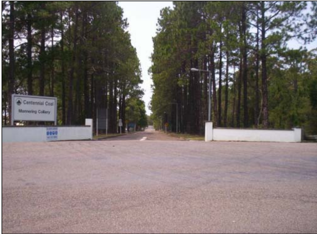
Photo 1: Mannering Colliery Access Road
