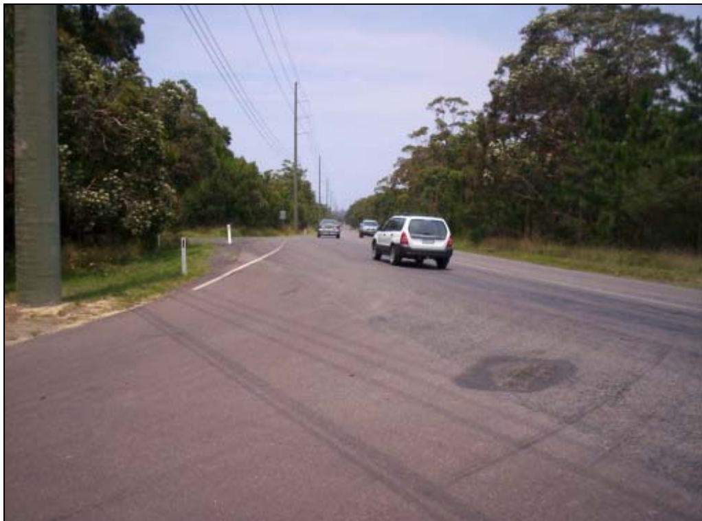
Photo 4: Rutleys Road Southbound
