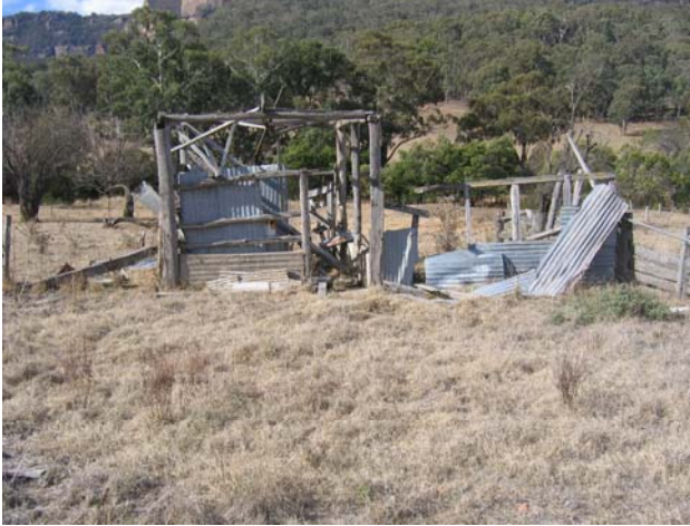
Figure 3.21: Remains of Slaughterhouse
