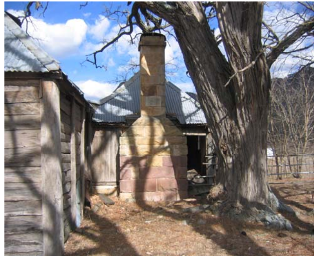
Figure 3.10: North Elevation of North-South wing showing chimney
