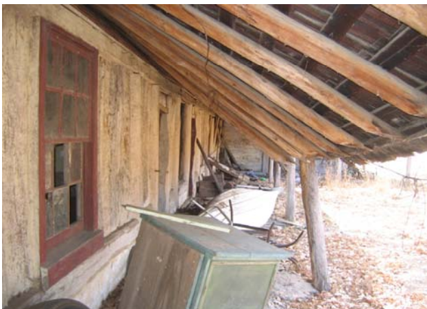
Figure 3.13: East Elevation showing verandah
