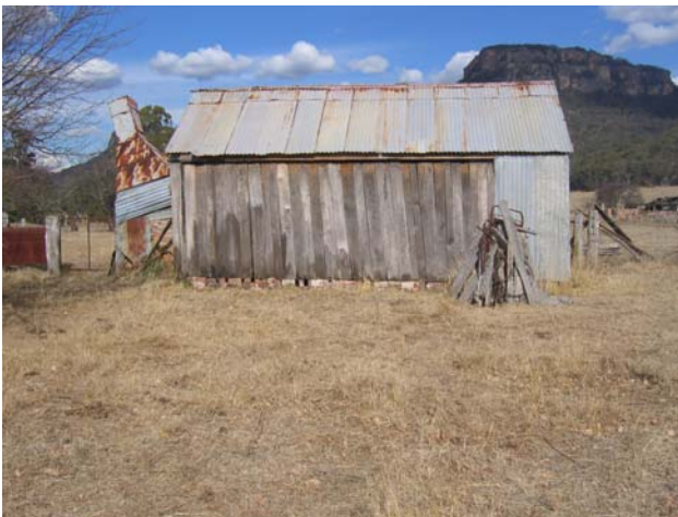
Figure 3.17: North Elevation of Men's Quarters
