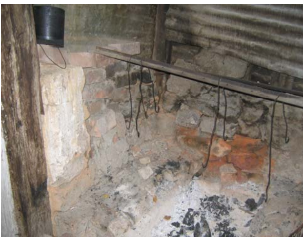
Figure 3.19 Interior of Men's Quarters showing the Fireplace
