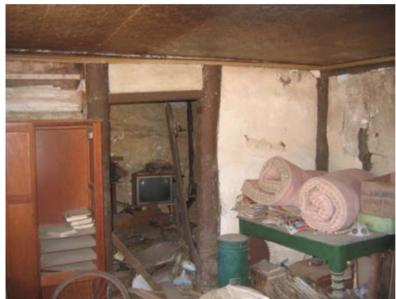
Figure 3.14: Interior of south room looking north
