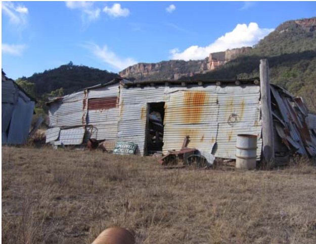
Figure 3.33: West Elevation of Barn
