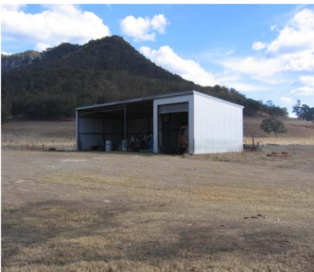
Figure 3.25 Prefabricated Farm Shed
