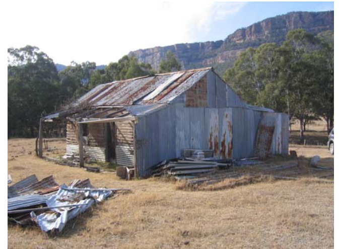
Figure 3.36: South and West Elevation of Timber Lathe and Mud Hut
