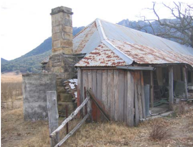
Figure 3.5: West Elevation of homestead showing Kitchen Chimney
