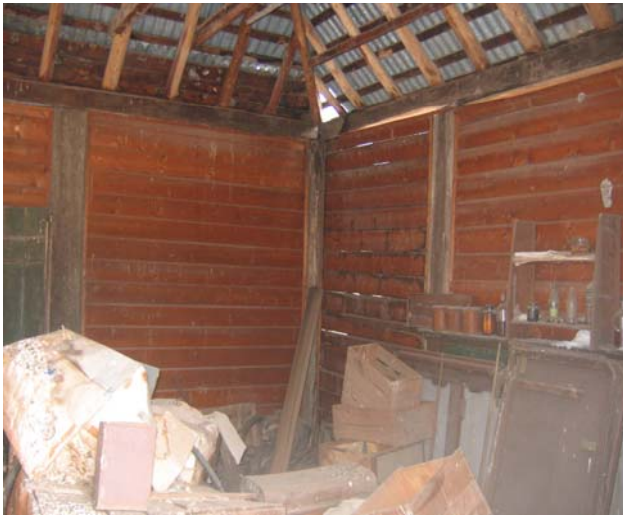
Figure 3.9: Interior of East-West Wing showing exposed rafters and corrugated metal sheeting
