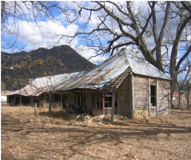
Figure 3.3: East and North Elevations of homestead
