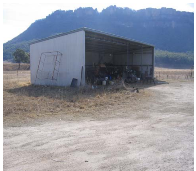
Figure 3.26 Prefabricated Farm Shed
