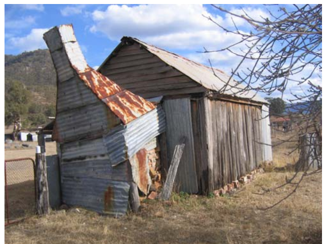
Figure 3.20 Worker's Hut from the north east
