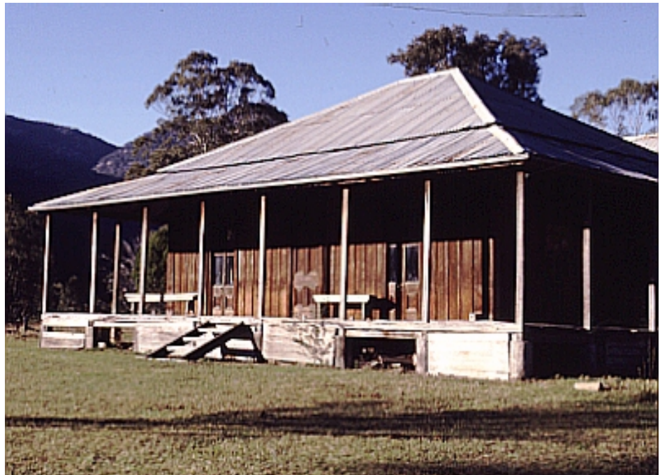
Figure 3.40: Kunderang East Homestead (Source: NSW Heritage Office, State Heritage Register Listing)
