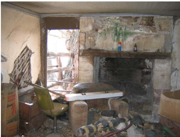
Figure 3.11: Interior of homestead showing stone chimney, painted lathe plaster walls and pressed metal ceiling.
