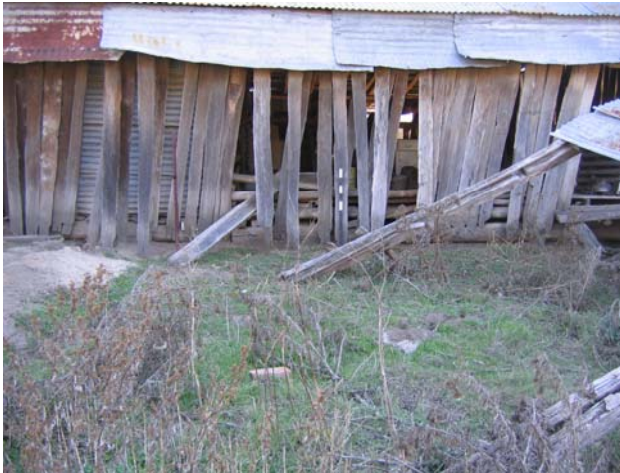
Figure 3.29: Part of North Elevation of Shearing Shed
