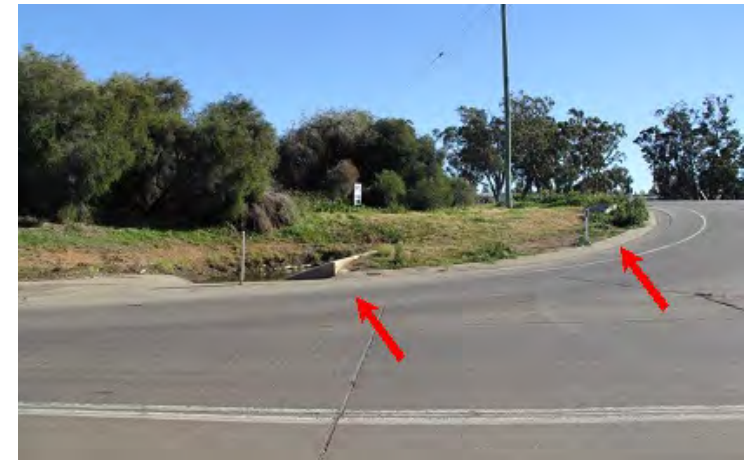
PLATE 7: Recommendation 7 Intersection of Quia Road and Torrens Road Note two unprotected culvert headwalls close to the edge of the carriageway.
