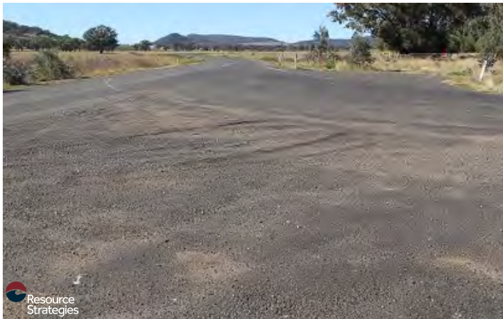
PLATE A3: Recommendation E Intersection of Coochooboonah Lane and Sunnyside Access Looking East Poor road surface and non-standard line marking. Double centre lines on Coochooboonah Lane through the intersection have been removed but remain visible.
