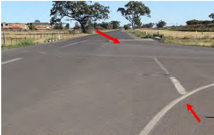
PLATE 4: Recommendation 4 West Along Quia Road from Farrar Road (Ross Road) Intersection Non-standard "stop" line and no left turn arrows on left only lane.
