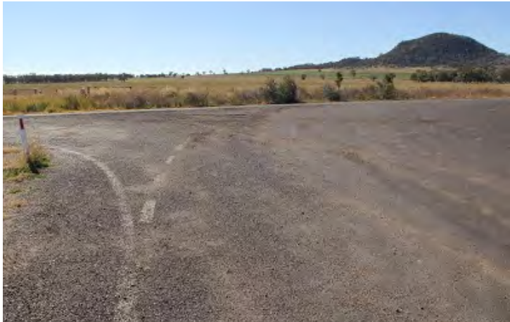
PLATE A1: Recommendation A Exiting from Sunnyside onto Coochooboonah Lane Poor road surface and non-standard line marking in poor condition.
