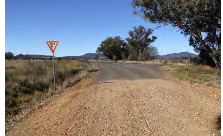
PLATE A2: Recommendation B Approaching Sunnyside Access Intersection from Coochooboonah Lane Southbound Give way sign approximately 25-30m in advance of intersection and no visible give way line for traffic approaching from Coochooboonah Lane southbound.
