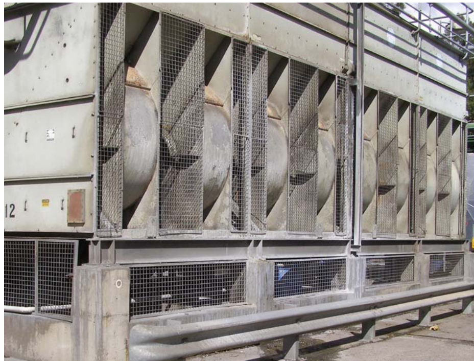
Figure 7 Existing Ammonia Refrigeration Plant (Evaporative Condenser)
