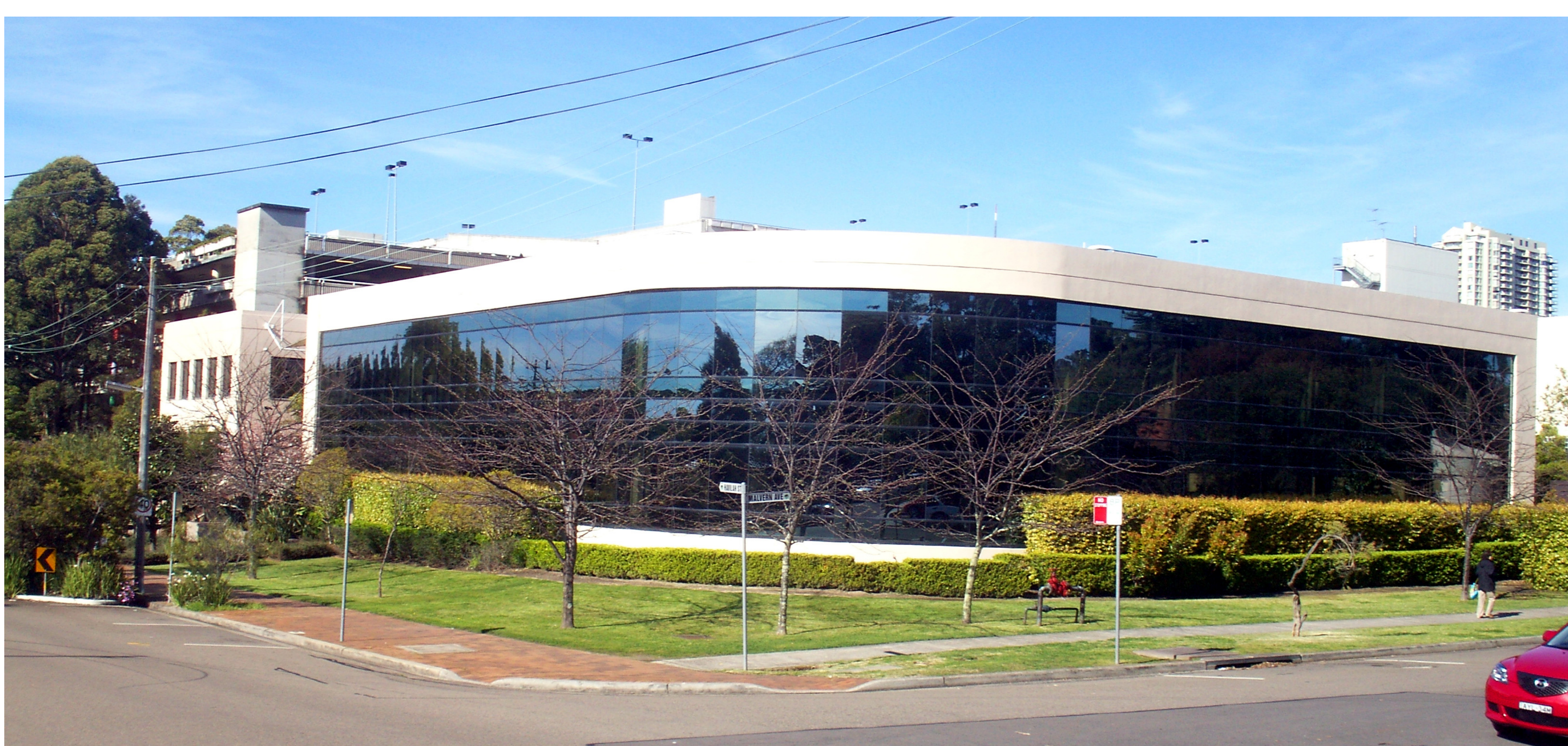
EXISTING STREETScape - CORNER HAVILAH ST & MALVERN AVE
