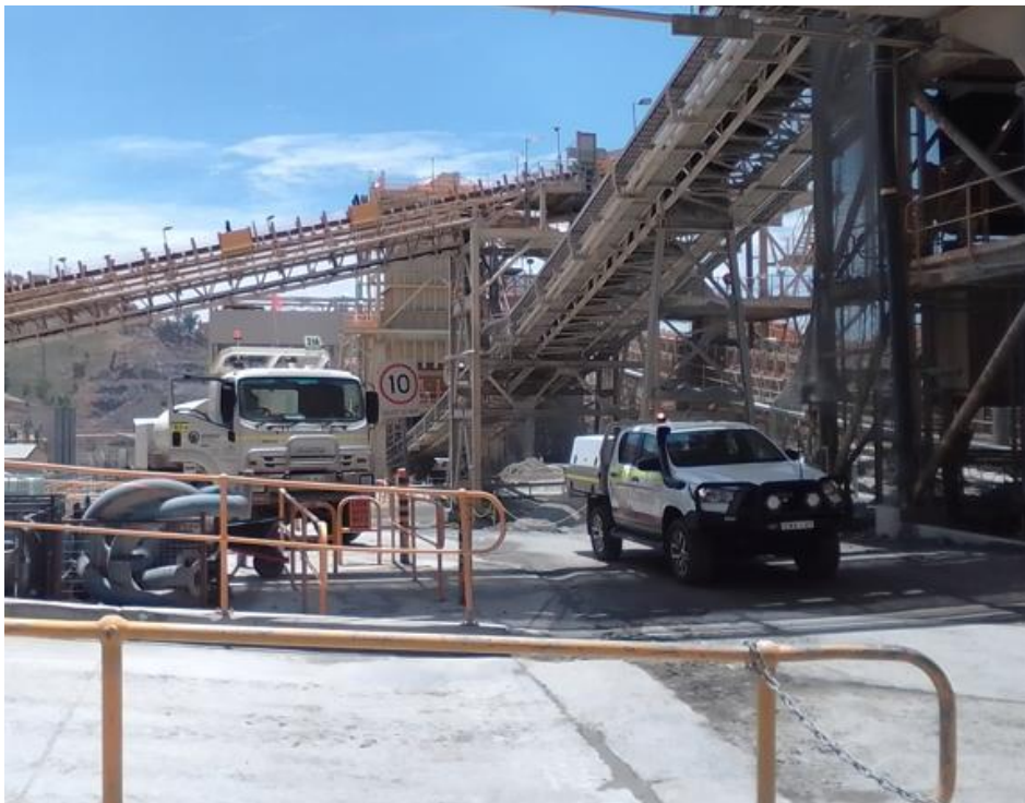
Plate 24 Speed limit signage in place within the mill area
