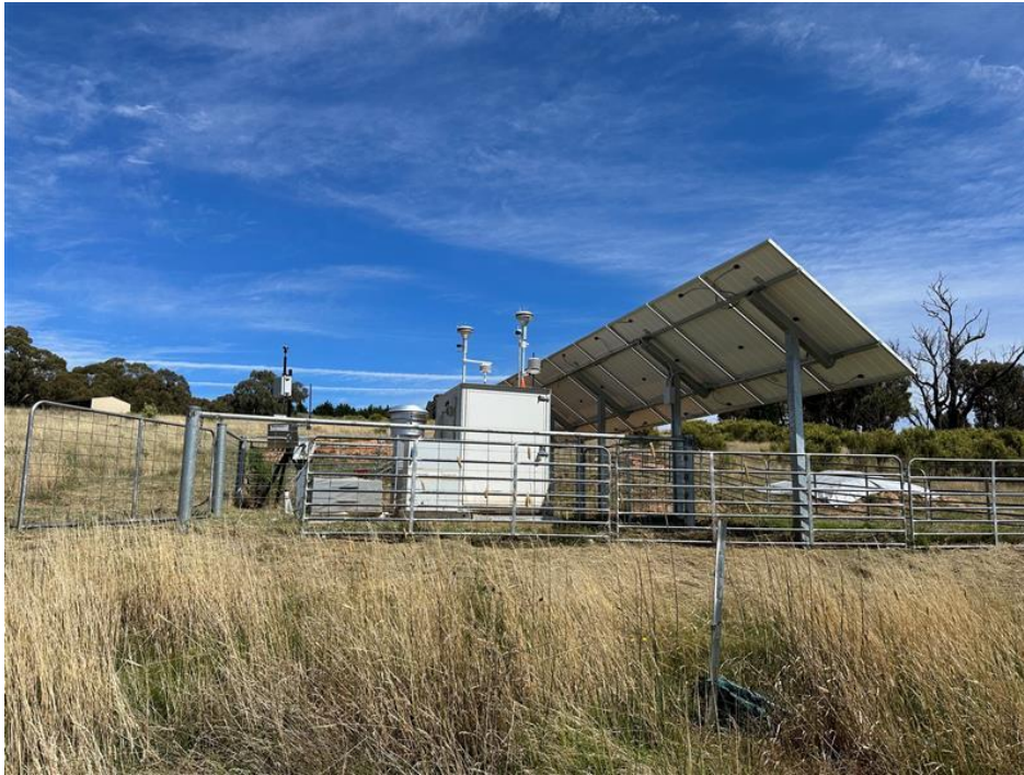
Plate 23 Woodville BAM site compound
