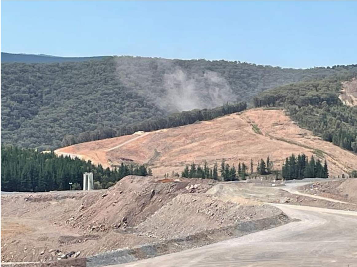
Plate 6 Visible dust emissions at site inspection (vegetation clearing within Cadia East Subsidence Zone)
