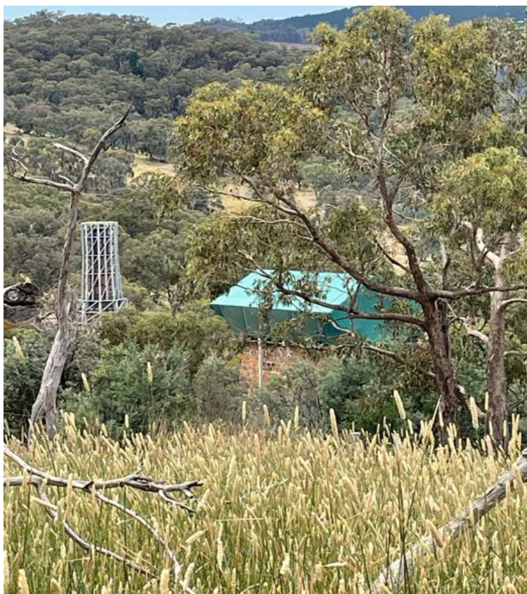
Plate 4 Cadia Cornish Engine house and chimney precinct (SHR0079)
