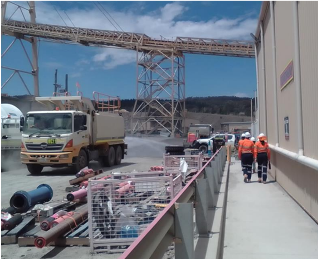
Plate 15 Water cart operating for dust control at the mill area
