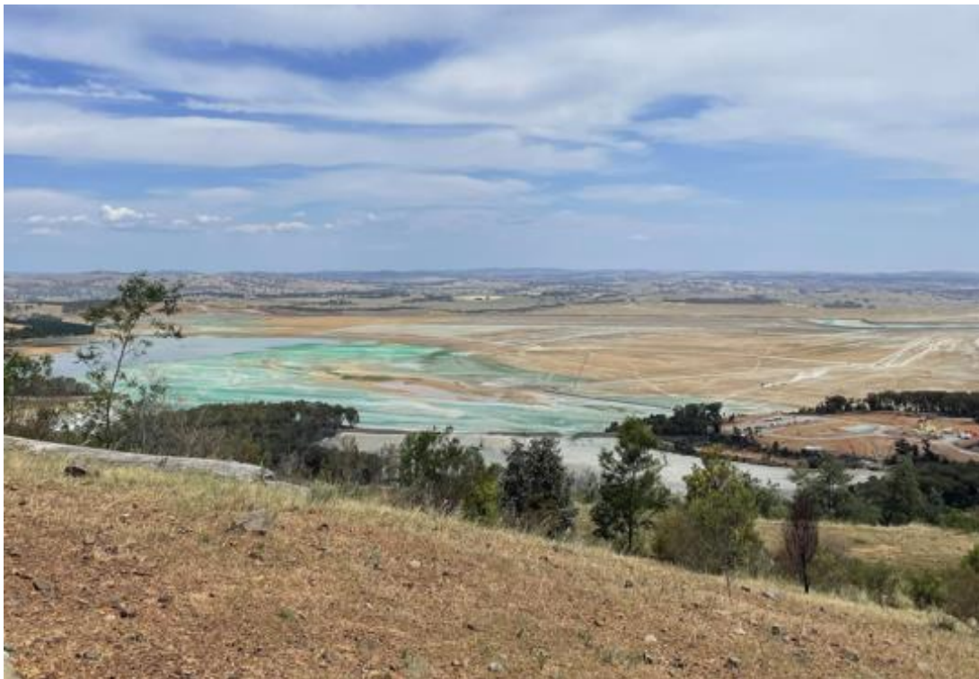
Plate 20 Tailings Storage Facility which has undergone aerial spraying to minimise dust lift-off
