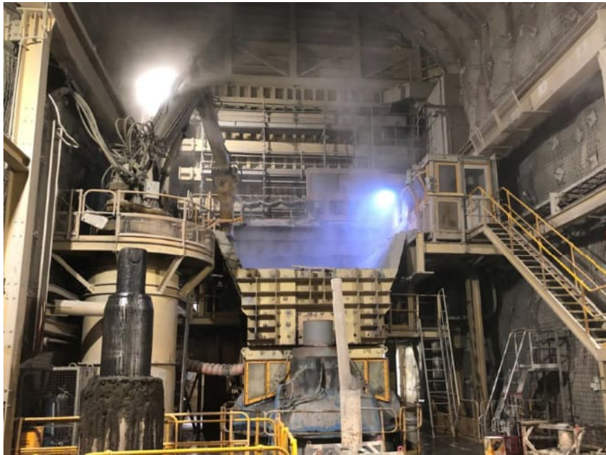
Figure 24 Typical Dust at PC1 Crusher Station
