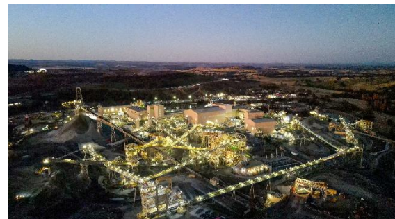
Plate 1-1 Cadia Ore Processing Facilities
