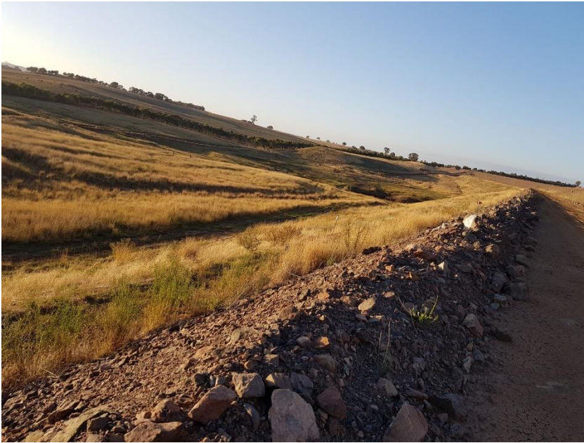
Plate A7-1: Eastern buttress area looking south. No trees
