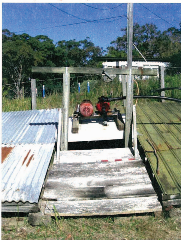
View of the exterior of the mine shaft showing timber platform, bearers and water pump (looking south).
