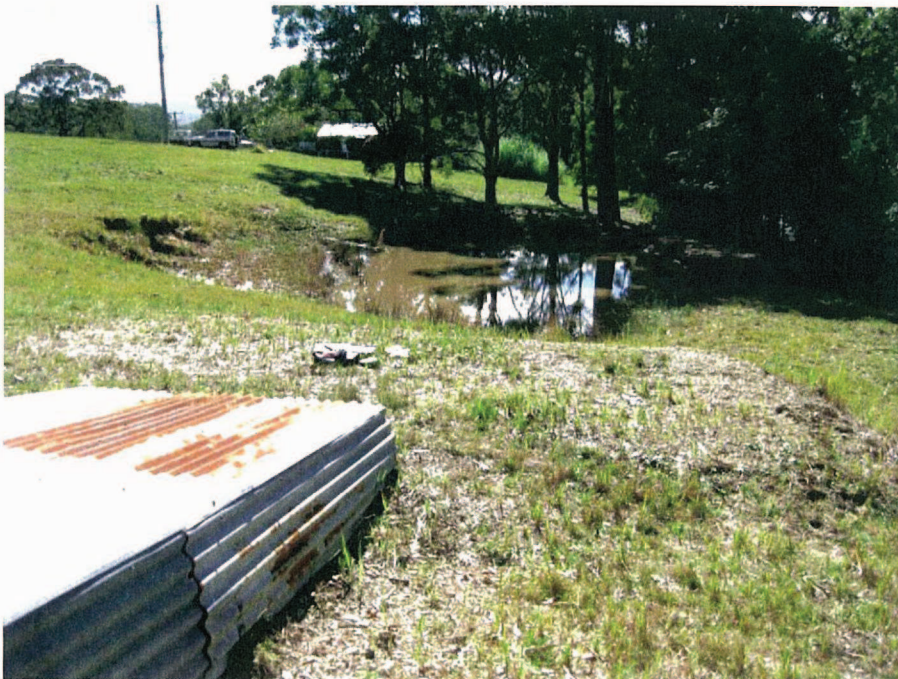
View of dam in the background and skree and mining mulloch in the foreground. Metal platform covering the exterior of the mine shaft in bottom left hand corner of the image (looking north).
