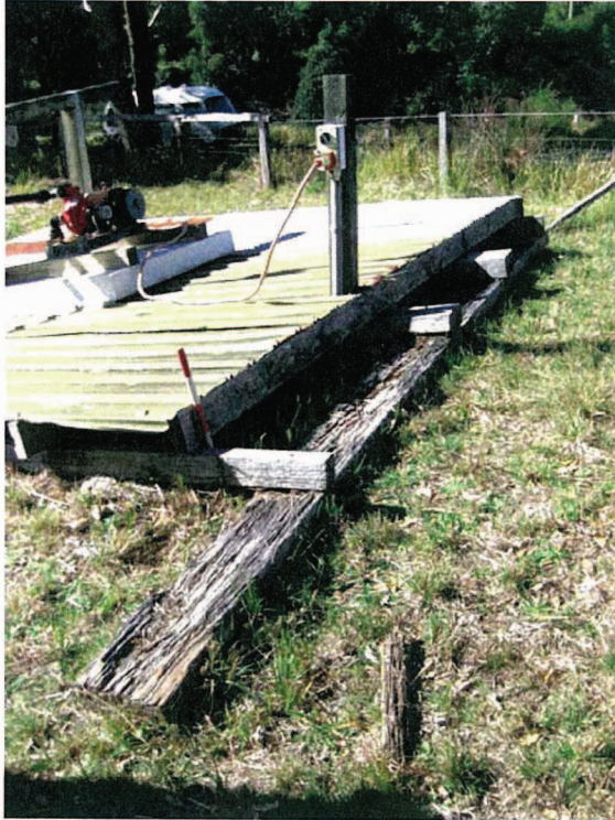
Exterior of the mine shaft showing timber bearers on the western side of the platform (looking south east).
