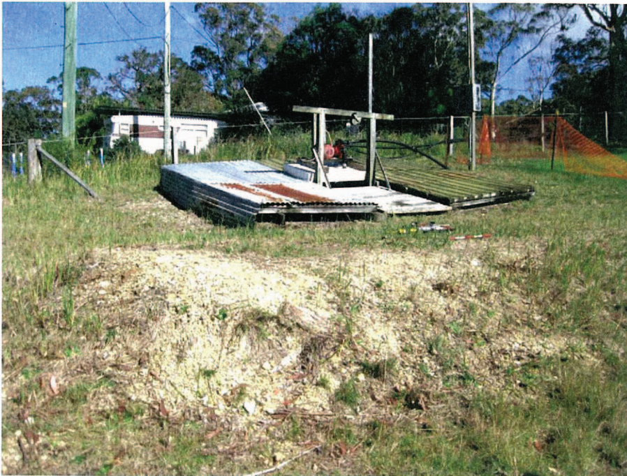
View of exterior of mine shaft (looking south-west) covered by timber and metal platform with water pump. Note skree and mining mulloch visible in foreground.
