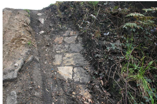
Plate 6: Sandstone retaining wall at the upstream Appin approach, facing north.
