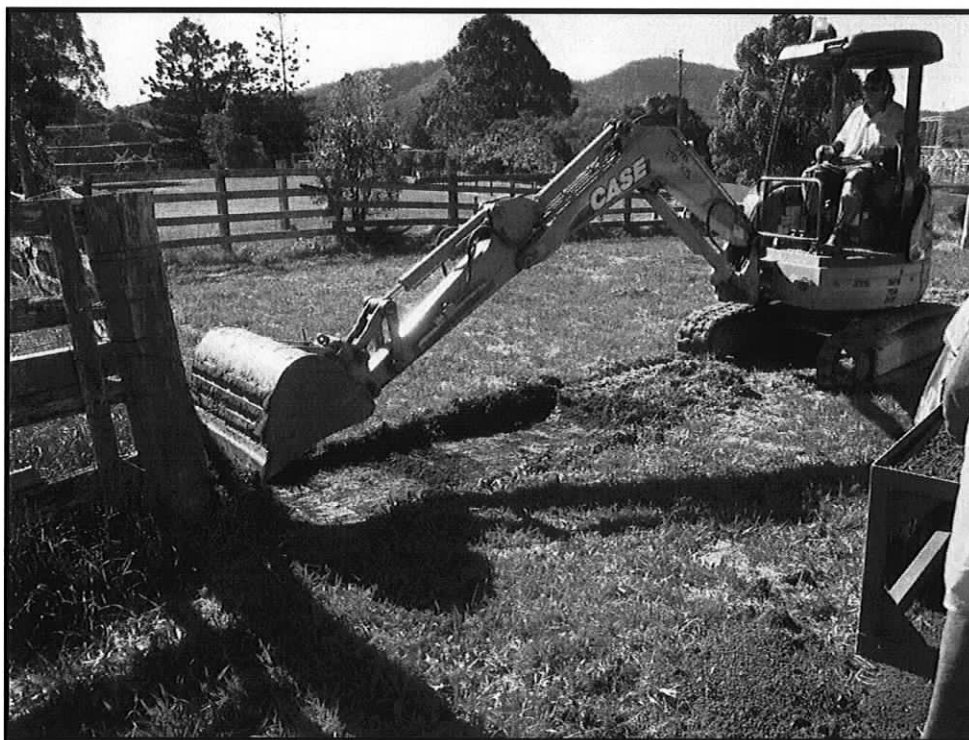
Plate 4. Typical excavation procedure (TP A2)
