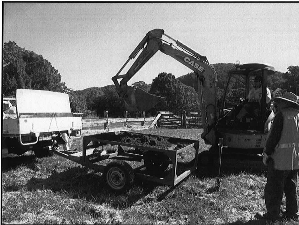
Plate 5. Excavated spoil placed directly on sieve (TP A3)
