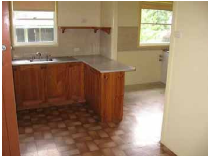
Photograph 7: Interior of house, 'wet area' walls consisting of cement fibre sheeting.
