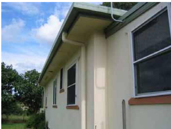
Photograph 6: Northern exterior of house with cement fibre cladding on exterior walls and eaves.
