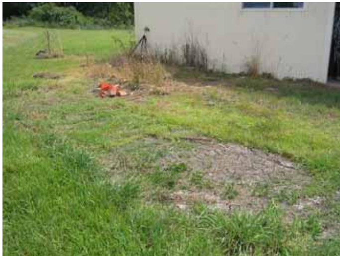
Photograph 5: Earth adjacent to garage / shed that appears to be old foot print of previous shed structure.
