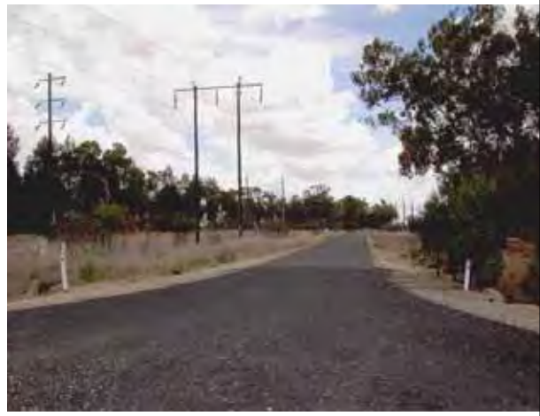
Photo Location 4 – View south from access road to existing substation and power plant site beyond. Parkes Peaking Power Plant screened by existing tree planting around substation site
