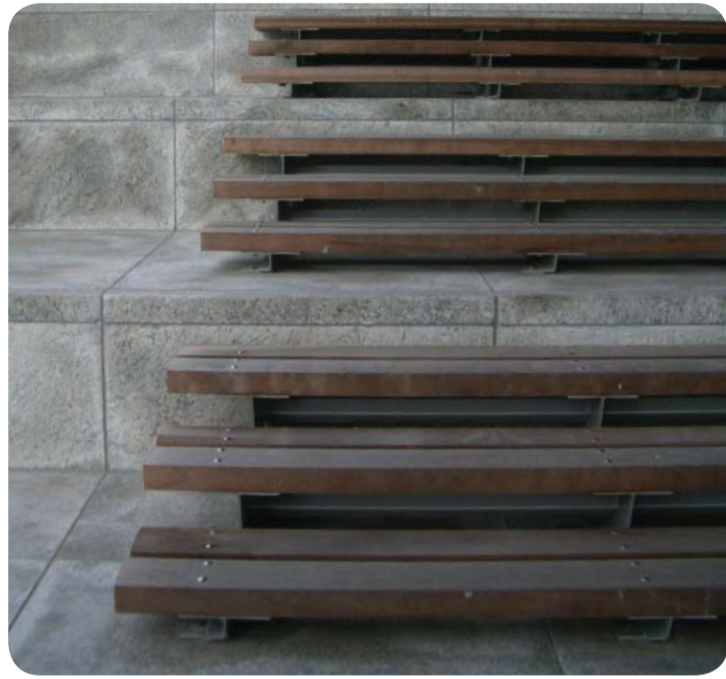
Timber stairs ASPECT Image Library
