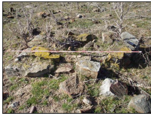
Figure 7.12 View west to collapsed stone chimney (Feature 4)
