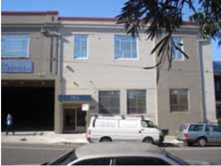
George St Buildings opposite NIDC site
