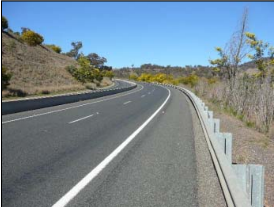
Photo 1 - View south along the New England Highway adjacent to the intersection with Quarry Road. Note sealed shoulder to both sides.
