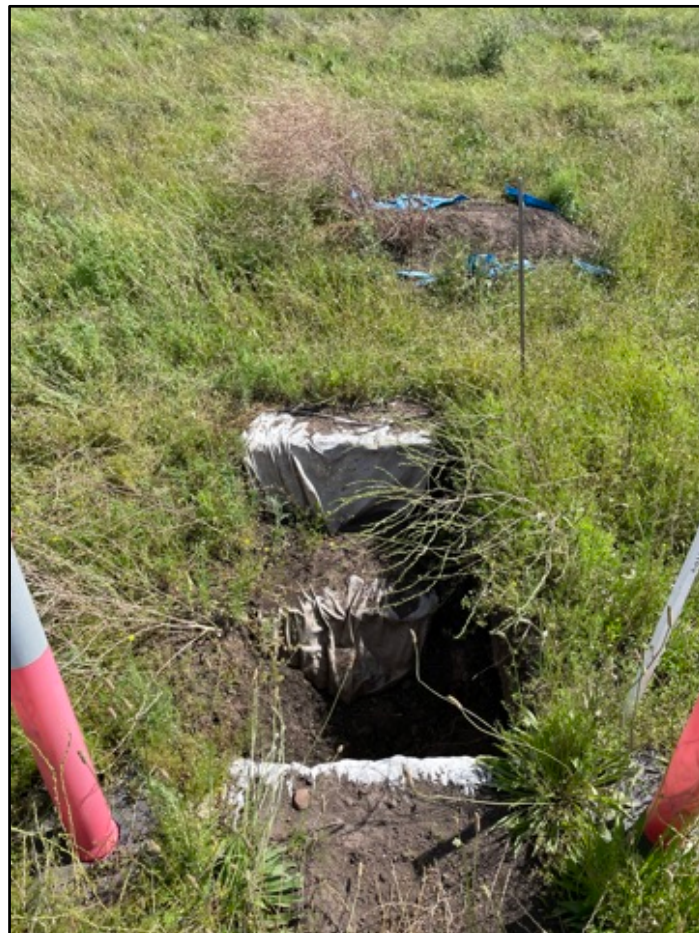
Open excavation pit within CM-CD1.
