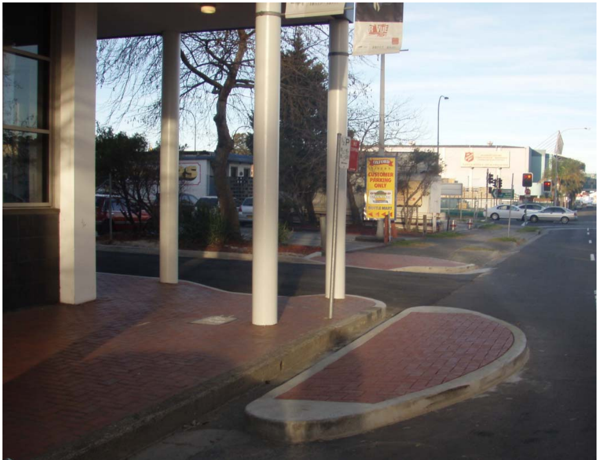
Figure 3 The support structures for the Wollongong Arts Centre and the kerb blister
