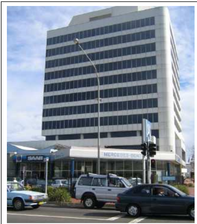
Figure 11 - Council administration building
