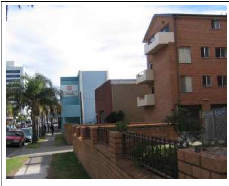
Figure 7 – Four storey residential flat building to the right of the picture
