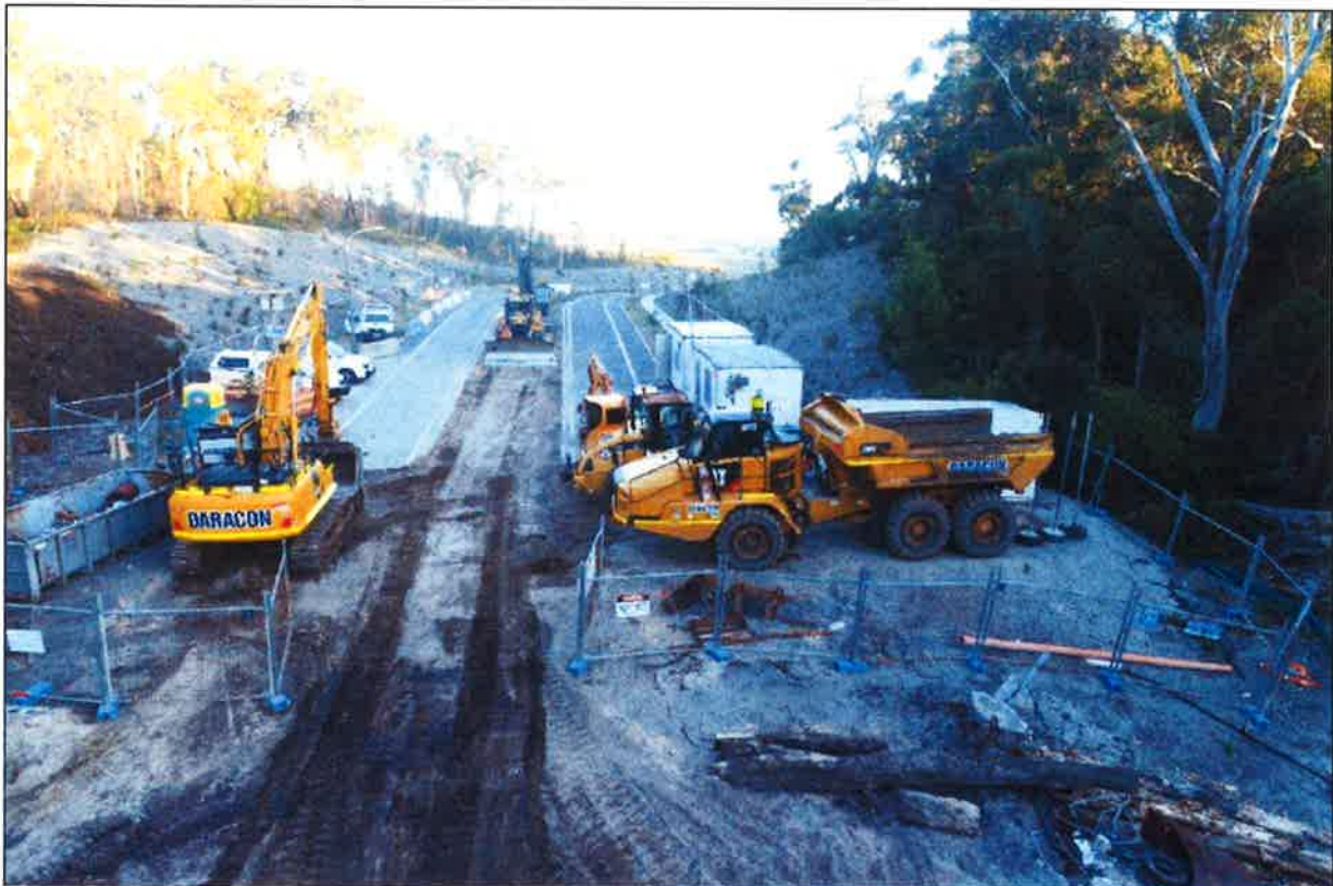
Figure 4| Construction of the Seaside Boulevard and Nelson Bay Road (Source: Applicant)
