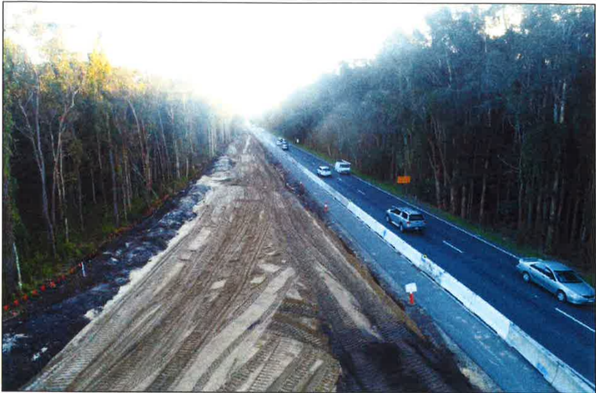
Figure 3| Construction looking south-west along Nelson Bay Road (Source: Applicant)
