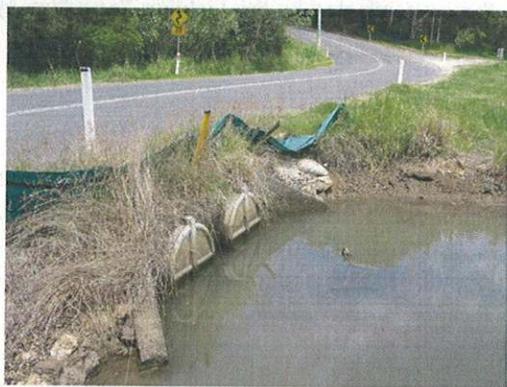
Figure 8: Stormwater culverts under James Drive
