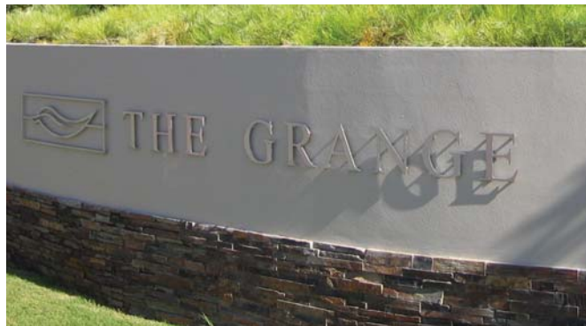
14) entry signage wall to consist of blockwork (semi-retaining) walls extending out of earth mounding with a painted and rendered finish. Lettering of subdivision name and possible logo to be pin fixed to wall to create shadows behind.
