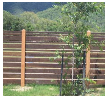
64) panels of timber fencing replicates the features in the entry to the site and breaks up long stretches of fencing
