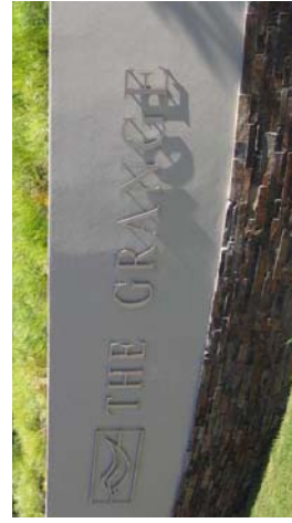
14) entry signage wall to consist of blockwork (semi-raining) walls extending out of earth mounding with a painted and rendered finish, lettering of subdivision name and possible logo to be painted to wall to create shadow effect to front
