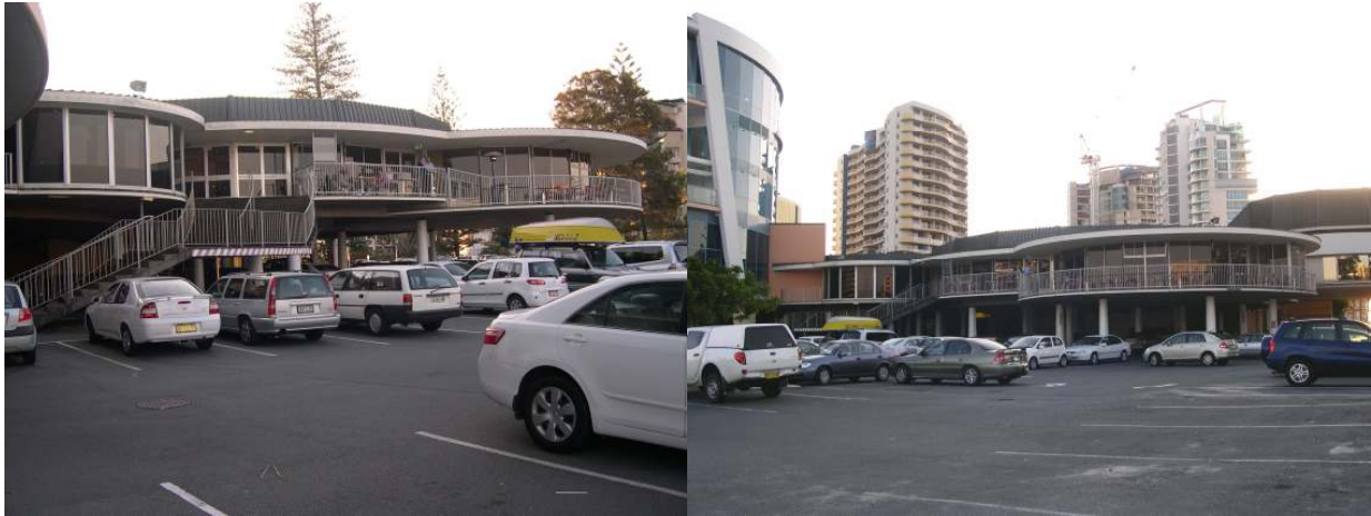
Figure 3: Two storey members building to be demolished as part of this application
