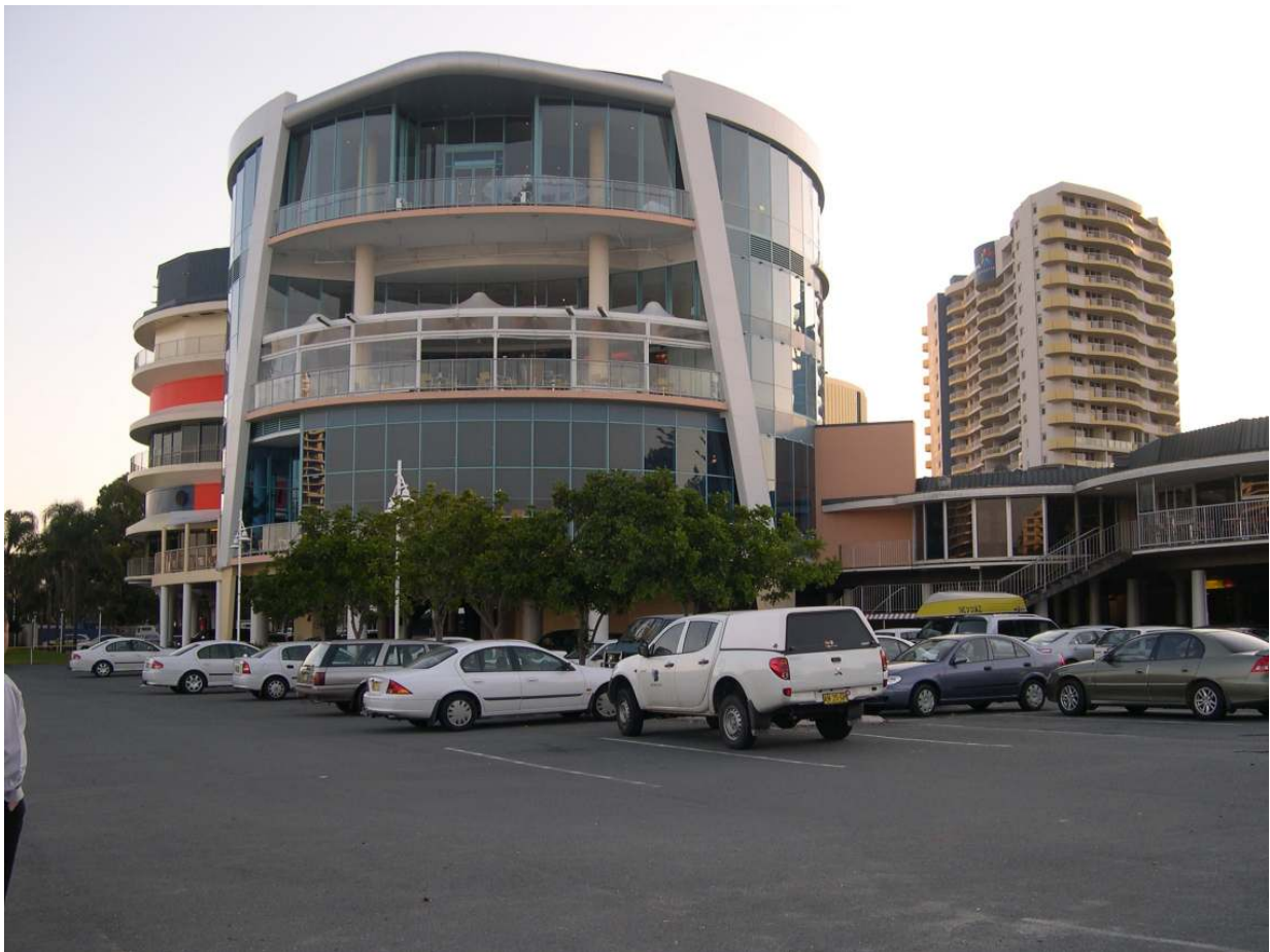
Figure 4: Millennium Building adjoining the proposed new building
