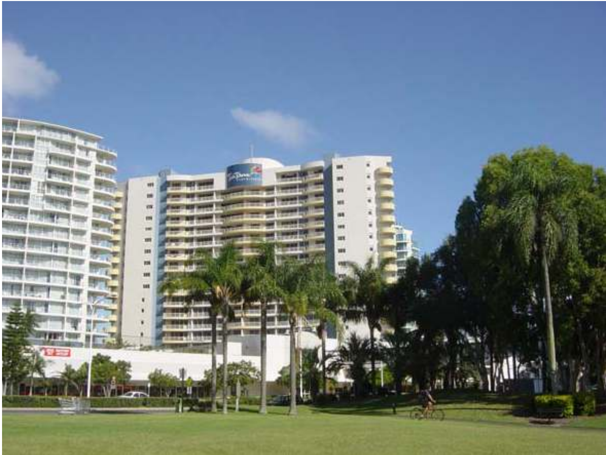
Figure 5: Twin Towns Resort Towers (Source: Environmental Assessment)
