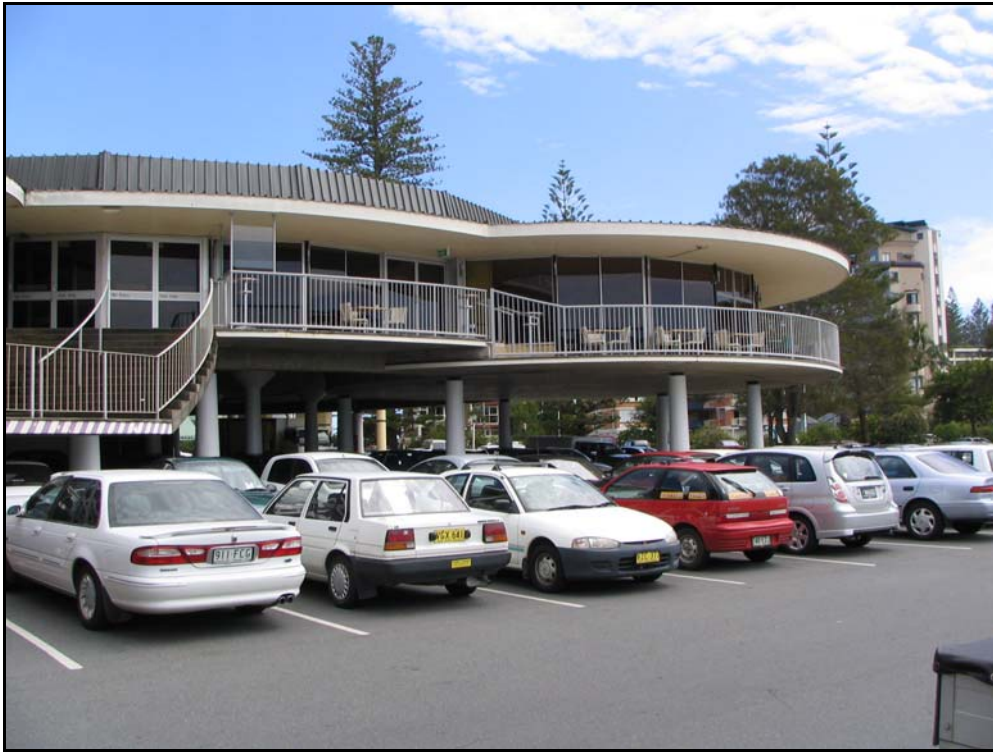
Photograph 1. View north to existing building.
