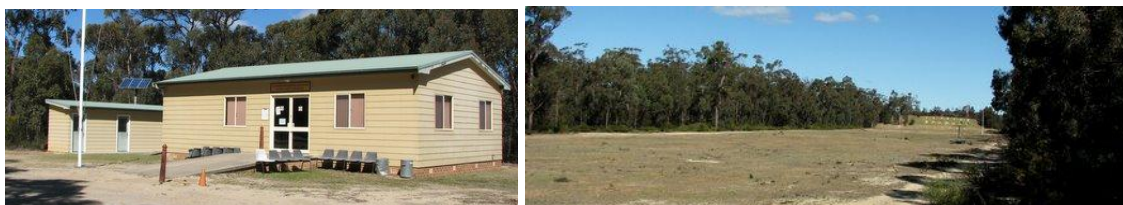
Figure 1-3 Eastern Club House Building and Amenities Block (L) and 800 m Shooting Range (R)
