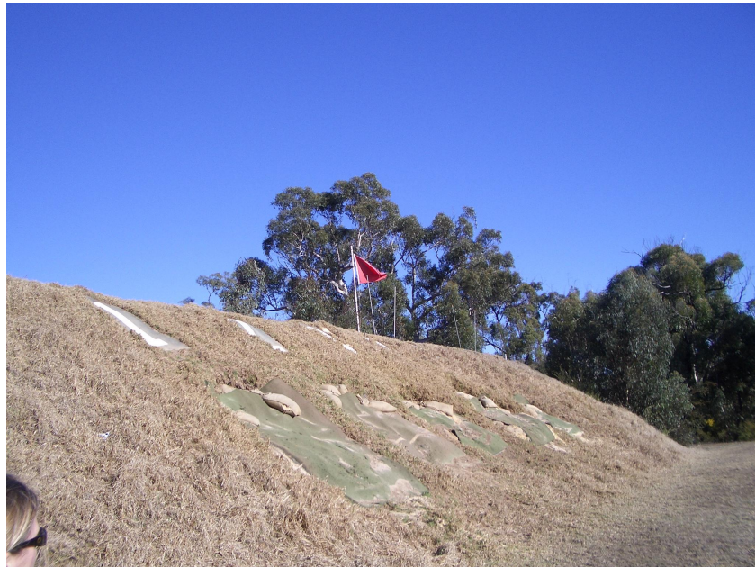
Figure 3.2 The existing rifle range stopbutt earth mound (located behind targets)
