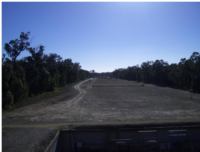
Figure 3.1 The existing 800m long rifle range (looking northeast) from the stopbutt
