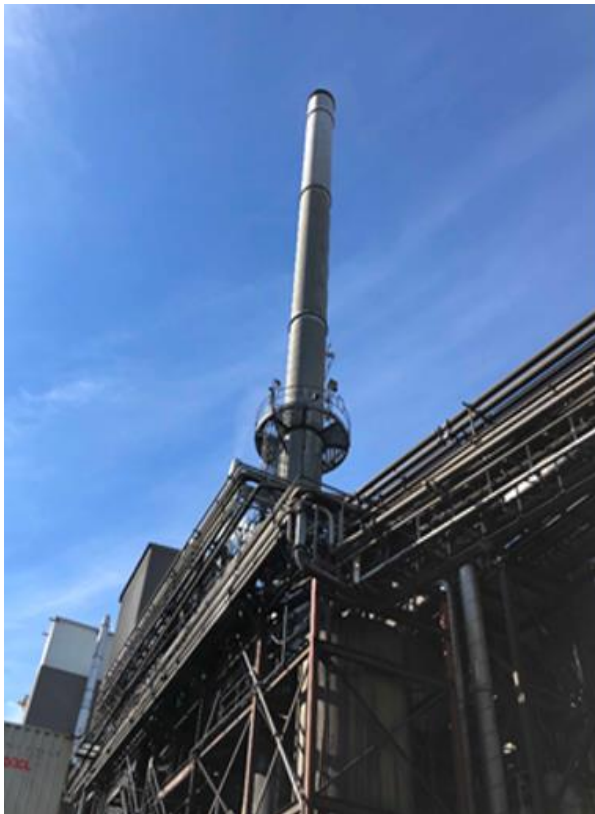
EPA ID 35 - Combined Boiler 5 & 6 Stack
