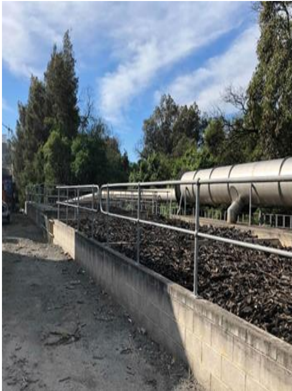
EPA ID 41 - Biofilter B
