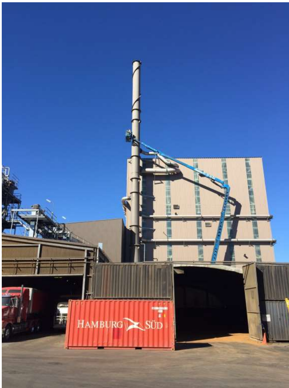
FIGURE D-29 DDG PELLET PLANT STACK – SAMPLE LOCATION PHOTOGRAPH
