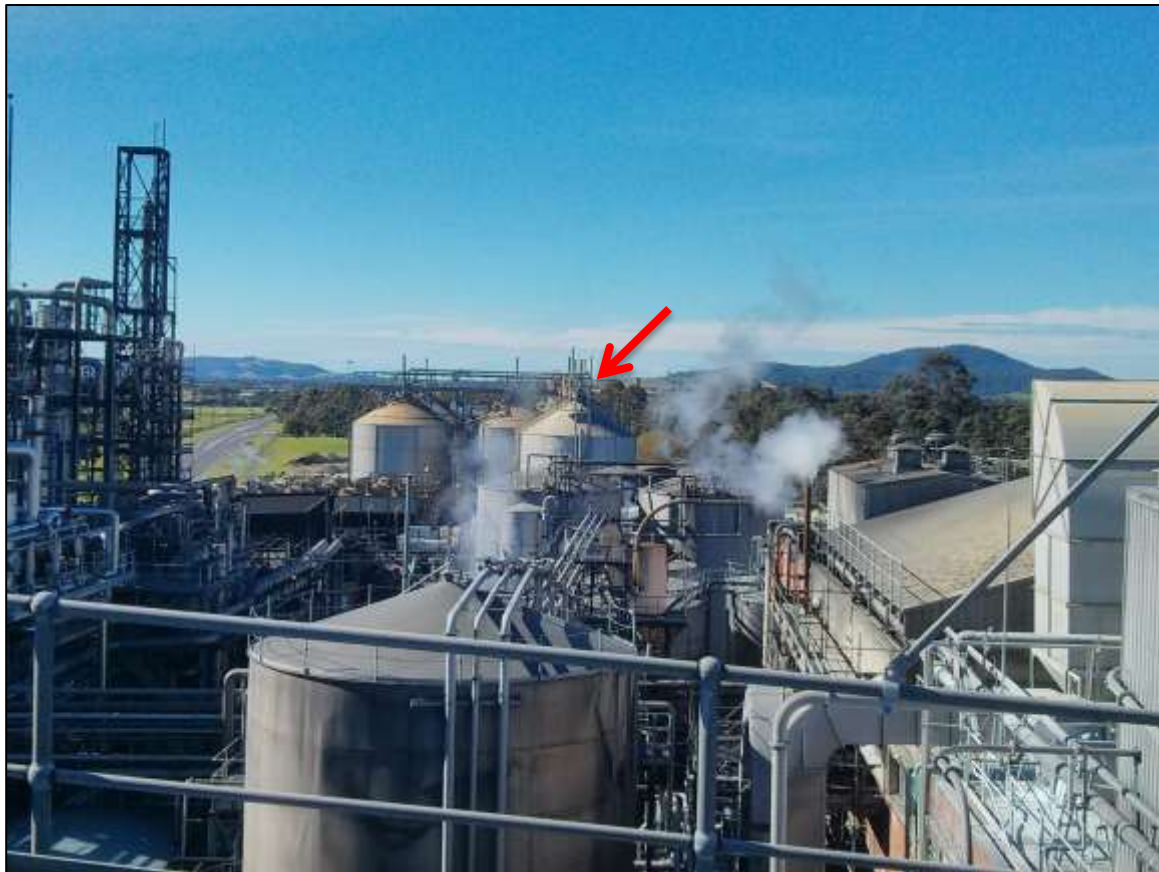
FIGURE D-18 FERMENTERS – SAMPLE LOCATION
