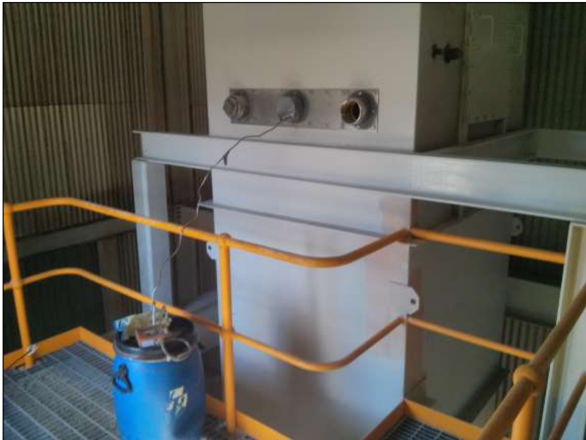
FIGURE D-8 GLUTEN DRYER NO. 4 – SAMPLE LOCATION
