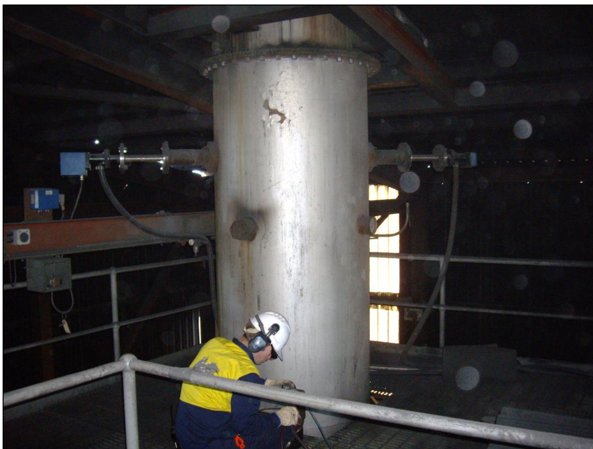
FIGURE D-23 BOILER NO 4 – SAMPLE LOCATION
